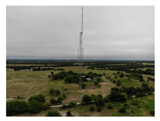
Tower is 180 feet AGL. The top antenna is 199 feet AGL and is the one being currently being used. The other two antennas are usable and available as backups in case the primary antenna fails. Ground elevation is 1140 feet AMSL.
