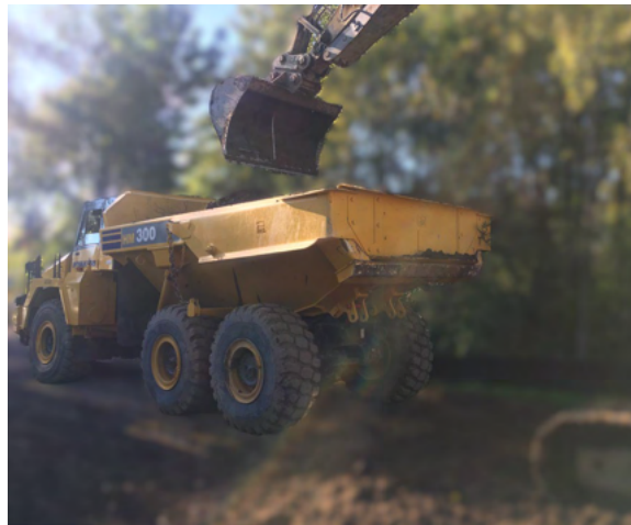
Exhibit 12. Off-road truck being loaded by excavator.
