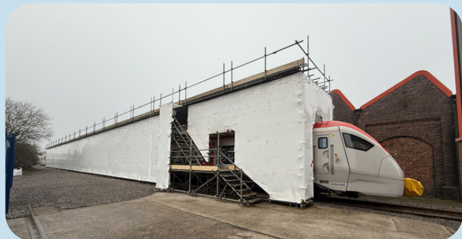
Barry Rail Depot enclosure, increasing maintenance capacity for the depot over busy periods.
