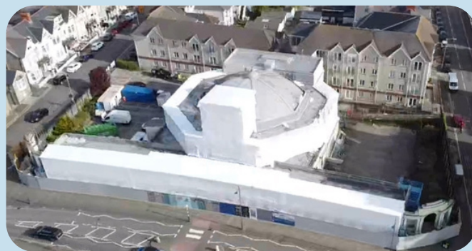
The Grand Pavilion, Porthcawl , enclosure allowed our client to blast the stone facade, while containing all debris.
