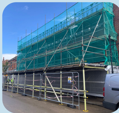
Burnham-On-Sea, High St , emergency repairs within the busy shopping precinct.
