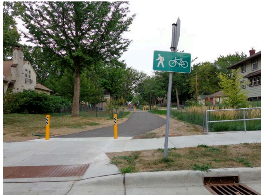
Figure 10 – 37 th Avenue North Greenway in Minneapolis. Constructed in 2011 by replacing a roadway with a trail and storm water gardens.
