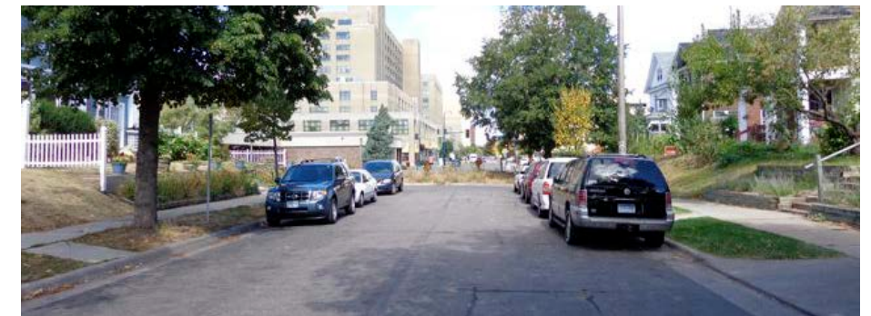
Figure 16 – Traffic diverter on 10th Avenue south of Lake Street, looking north.
