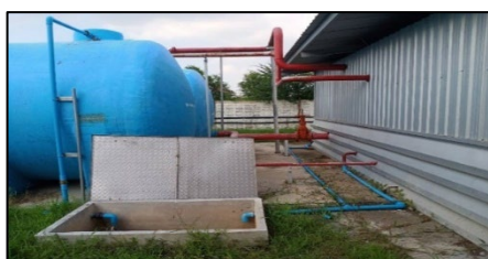
Water pipes directing water to the backup fire pump system
