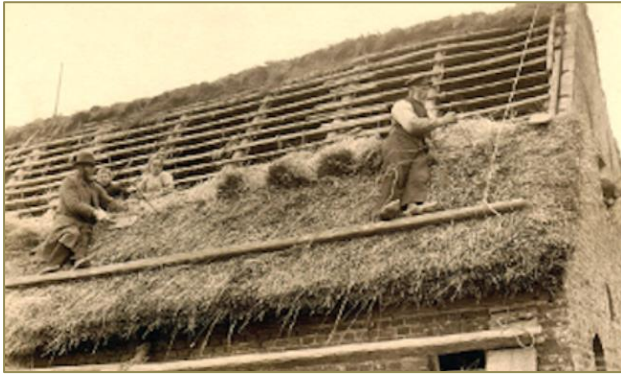
Thatching underway in 1914, showing the timber framing
