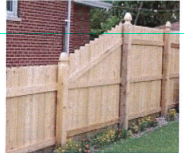
example of acceptable transition from 4' to 6'
