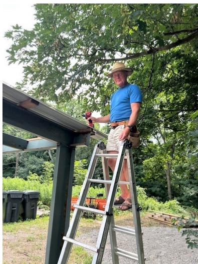
A cool cat on a hot tin roof... Dennis Kuhlmann putting on the final touches of Tim's new wood shed
