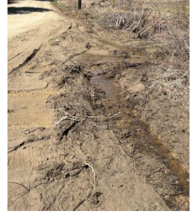
(Left) Culvert is slightly crushed. (Right) Bare soil and eroding road shoulder has caused a channelized path for stormwater.
