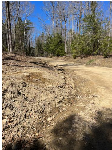
(Left) Road shoulder erosion and bare soil on Crest Road at the intersection of O'Neill Road. Consider if the bare soil area is a suitable site for a rain garden. (Right) Eroding ditch looking west, downhill on O'Neill Road.
