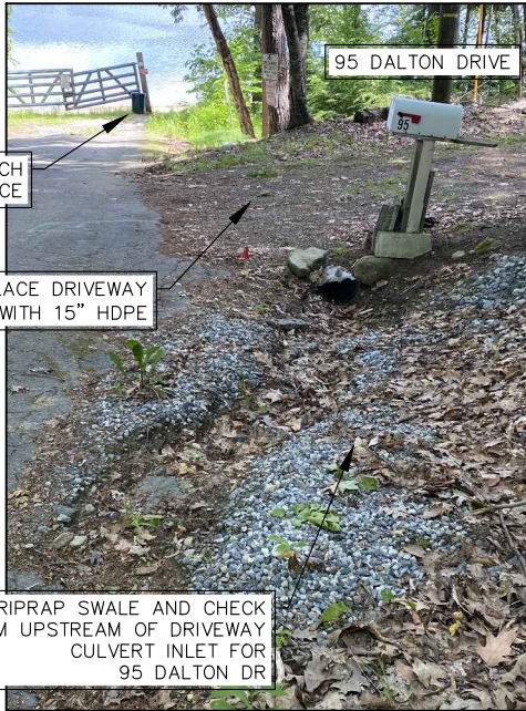
DALTON DRIVE DRAINAGE SWALE (EAST SIDE OF ROAD)
