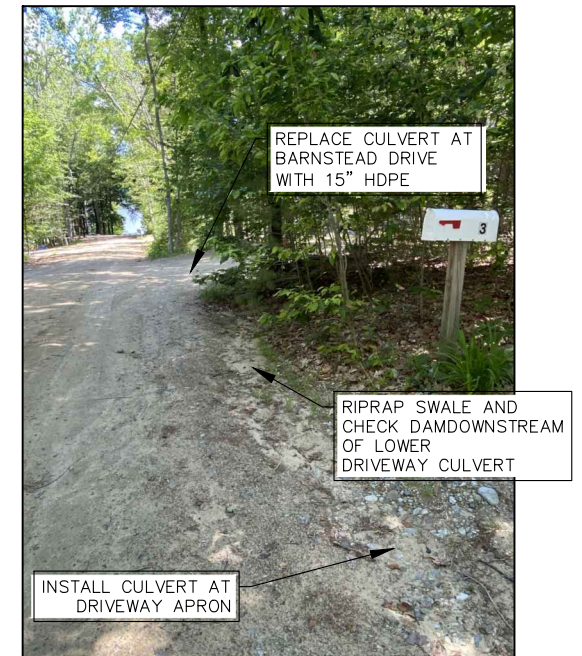
DALTON DRIVE DRAINAGE SWALE (EAST SIDE OF ROAD)
