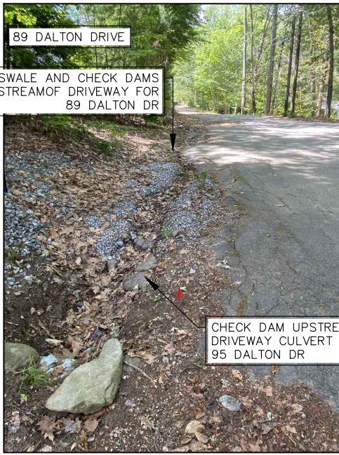
DALTON DRIVE DRAINAGE SWALE (EAST SIDE OF ROAD)
