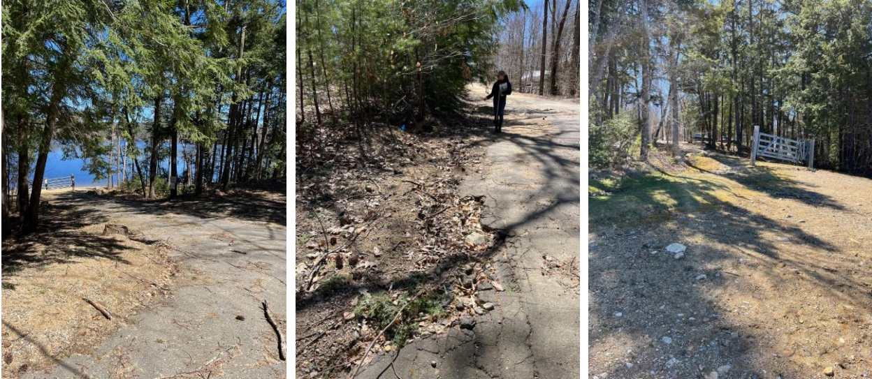
(Left) Road shoulder erosion on the side of the parking lot to the beach area. (Middle) Road shoulder erosion leading down from the parking lot. (Right) Gullies lead down from the road onto the beach and ultimately into the lake.
