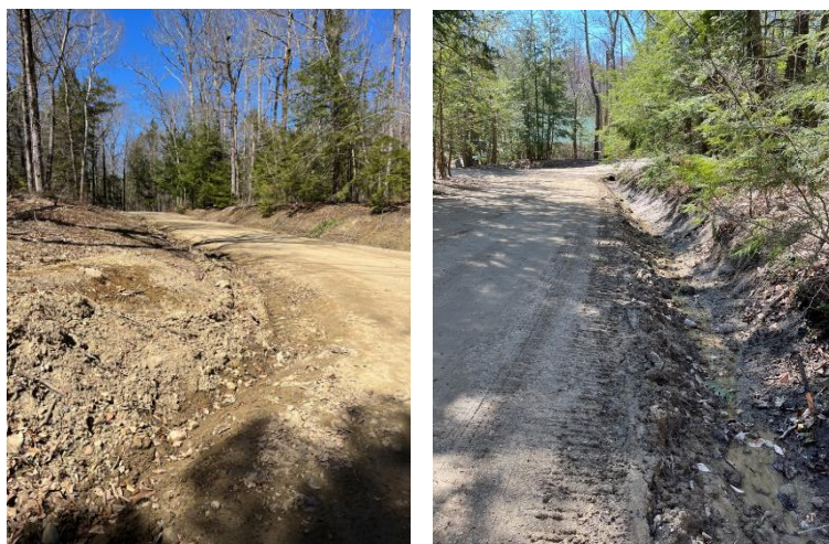
(Left) Road shoulder erosion and bare soil on Crest Road at the intersection of O'Neill Road. Consider if the bare soil area is a suitable site for a rain garden. (Right) Eroding ditch looking west, downhill on O'Neill Road.
