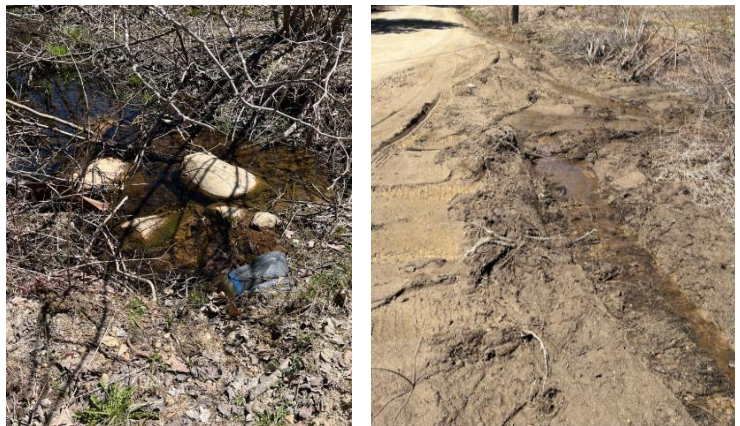
(Left) Culvert is slightly crushed. (Right) Bare soil and eroding road shoulder has caused a channelized path
