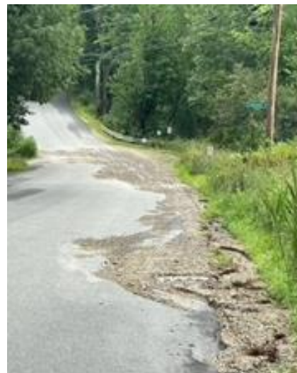
The eroding road shoulder leading to the North Barnstead Rd boat ramp.
