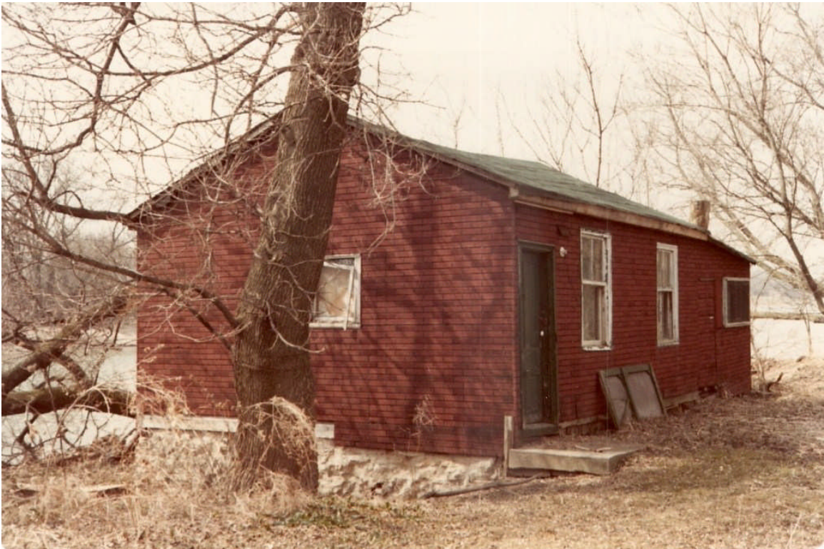
Structure at Abraham Young site (now demolished) – SE corner – March 1981
