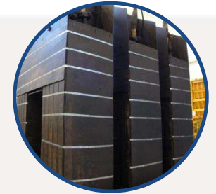
Transformer opening - before core removal
