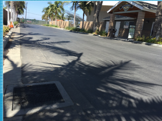
MALL AND GROUND PRESSURE WASHING Water bubbles out here, goes to gutter, flows off-site into storm drain
