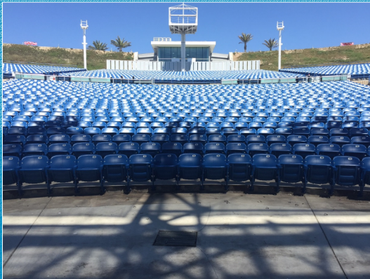
PACIFIC AMPHITHEATER PRESSURE WASHING Water drains here and gets pumped to Storm Drain
