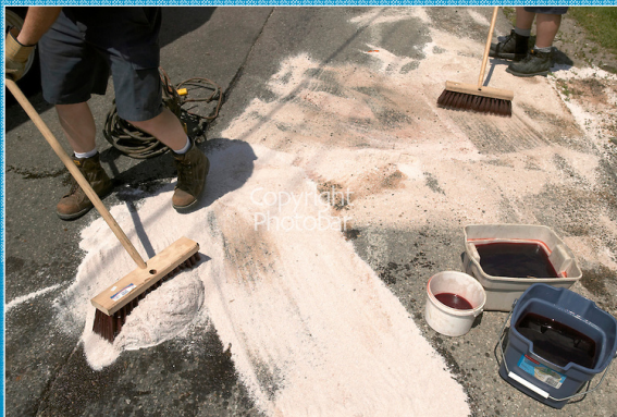
Non-hazardous OCFEC Internal Oil Spill Clean Up
