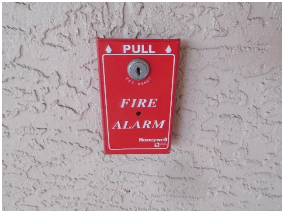
TYPICAL MANUAL FIRE ALARM
