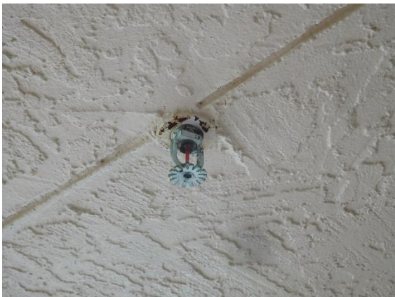
TYPICAL FIRE SPRINKLER HEAD
