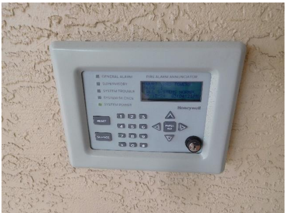
TYPICAL FIRE ALARM CONTROL PANEL
