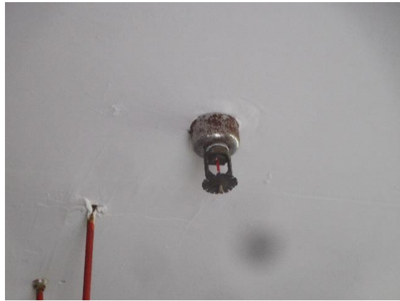
FIRE SPRINKLER HEAD PUMP HOUSE
