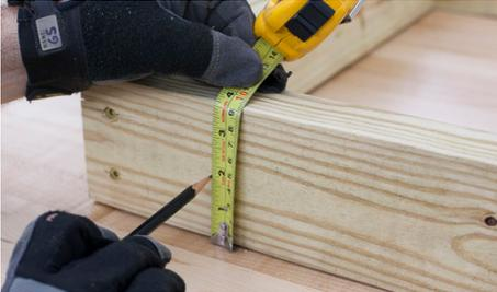
On the outside of part (A), mark a point 4" from the left edge and 1 3/4" from the top edge.
