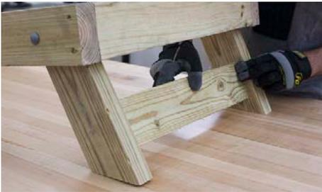
Position part (D) between parts (C), making sure that it is about an inch off the work surface.
