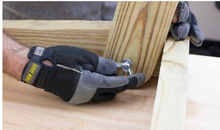
Install the washer and wingnut to secure the angled supports.
