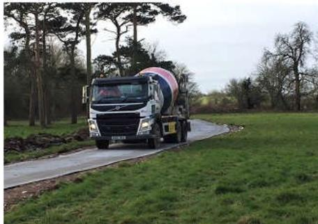
Initial works started in January, when the service access was made. Since then, the ground has been prepared and the drainage laid. This was followed by the delivery of the concrete for the foundations.
