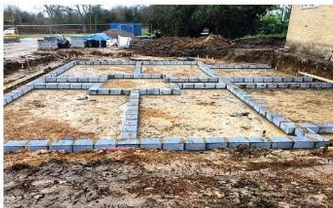
Next came the block work and from there the floor plan of the building really started to take shape. When this has been done, the timber framework will be fitted.
