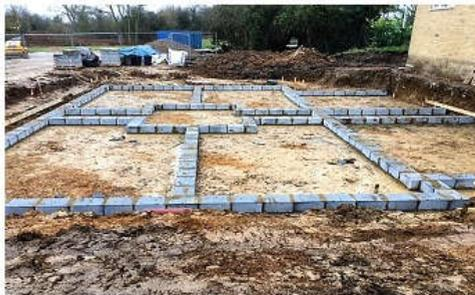
Next came the block work and from there the floor plan of the building really started to take shape. When this has been done, the timber framework will be fitted.
