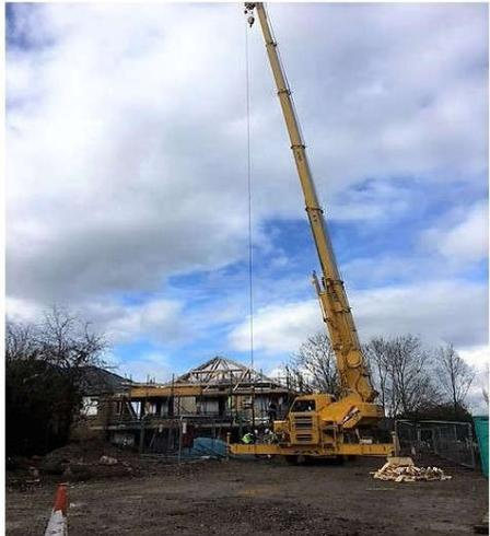
Whilst this was progressing, the plumbing work continued and the framework has been insulated and lined. Now the roof slates are going on and the building will soon be watertight ready for internal works to become the focus for the next stage.
