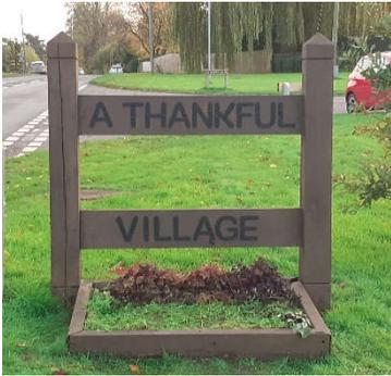
It is hoped that most of you will have by now have noticed the recent maintenance work carried out to the village entrance gates. The main uprights which were starting to rot through have been reinforced with new concrete repair posts. All woodwork has been treated with preservative/wood stain and the failing 'A Thankful Village' vinyl lettering has been removed and replaced with new rigid acrylic letters.
