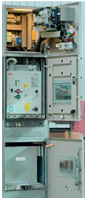
Figure 11: From top to bottom: Low voltage relay cabinet, medium voltage circuit breaker cabinet, voltage transformer cabinet.
