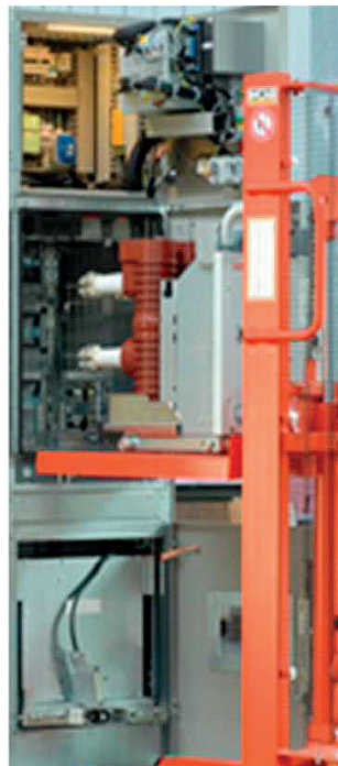
Figure 12: Shown with G&W VCB F circuit breaker withdrawn on cart.
