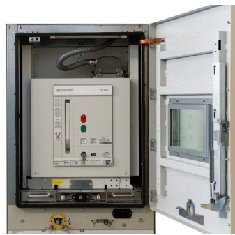
Figure 31: Withdrawable unit enclosure overall views, with unit installed
