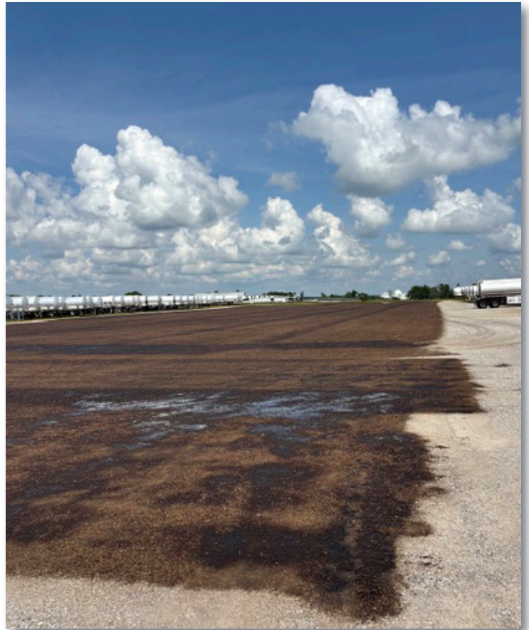
Construction project at Miller, MO, asphalt facility - new concrete pad (left) and dust control (below) in-house product applied with the help of Blevins Asphalt.
