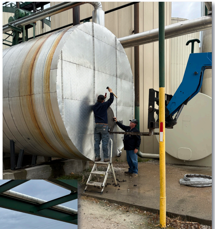
Construction project at Miller, MO, asphalt facility - Crews are decommissioning Tank 21 and removing piping in preparations to cut down three tanks and relocate Tank 21 (left and below).
