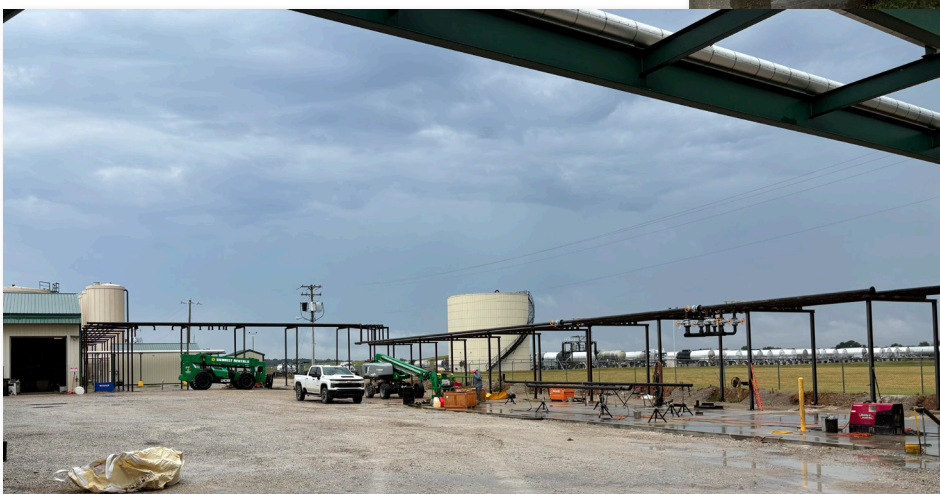
Construction project at Miller, MO, asphalt facility - new piping that is being put in to support the two new tanks as well as supply oil from the new hot oil unit (left).
