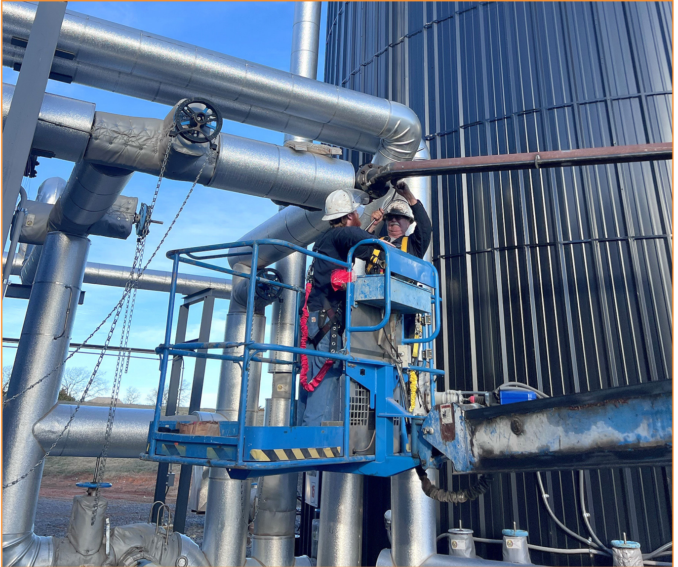
Ken Sasse and Robert Cline are pictured installing heat tracing on a new offload line at the Clinton facility.
