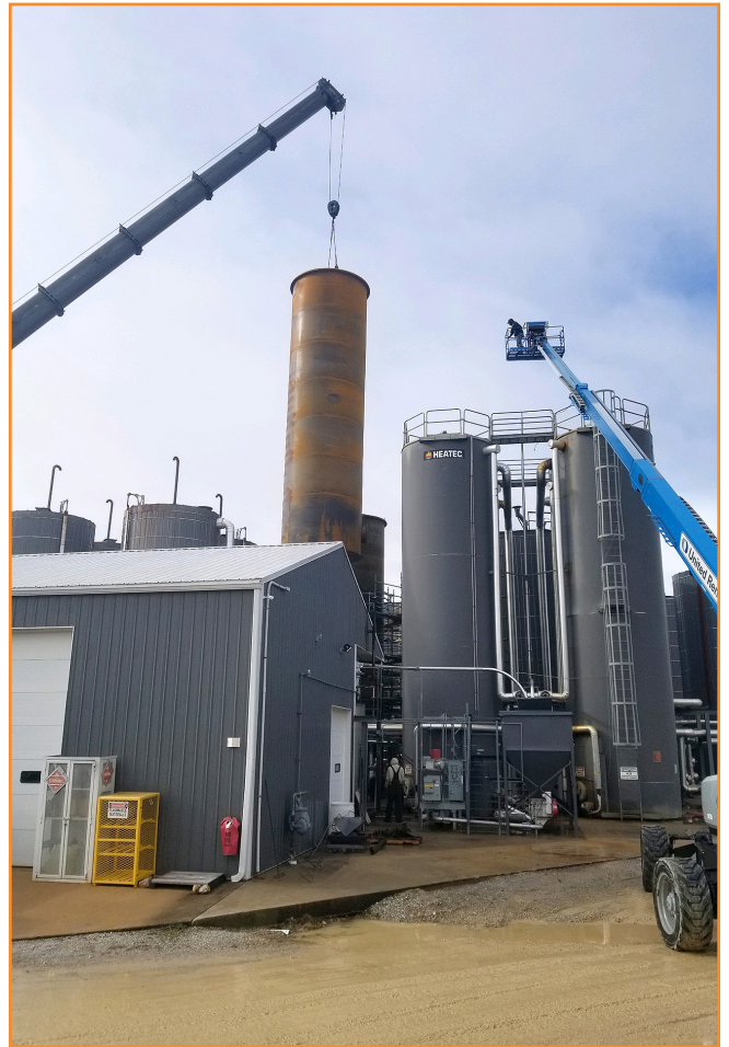
Eight new tanks have been set at the Willow Springs Rail Facility, replacing six that were removed late last year and two that had been removed previously.
