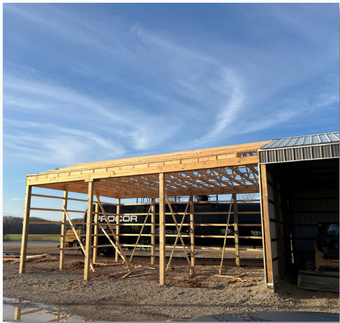
Additional equipment storage is being added at the Willow Springs Rail Facility
