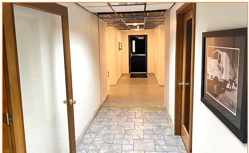
The hallway leading to the shop and the break room is shaping up.
