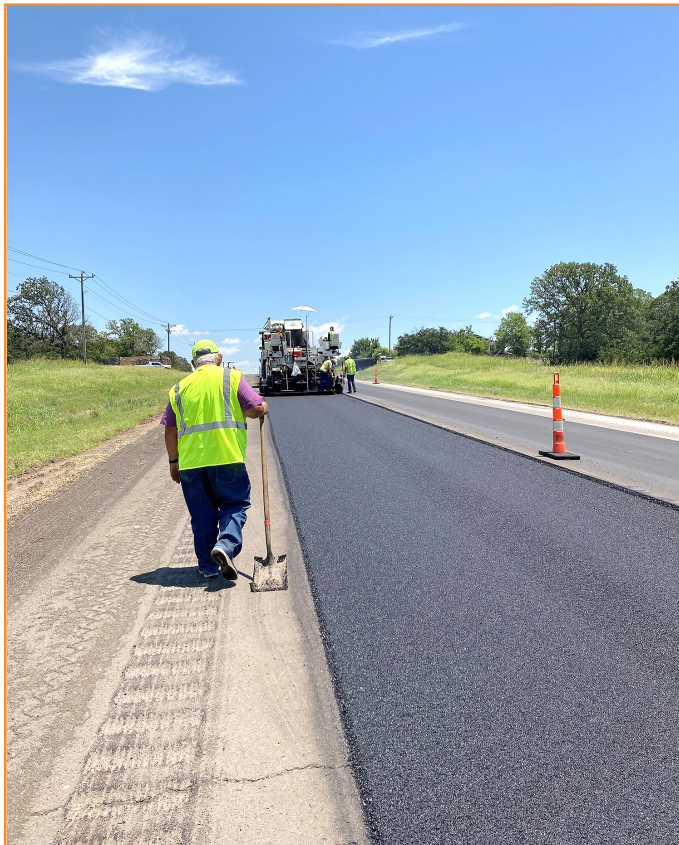
Pavers Inc. putting down 76-28E in Davis, Okla.
