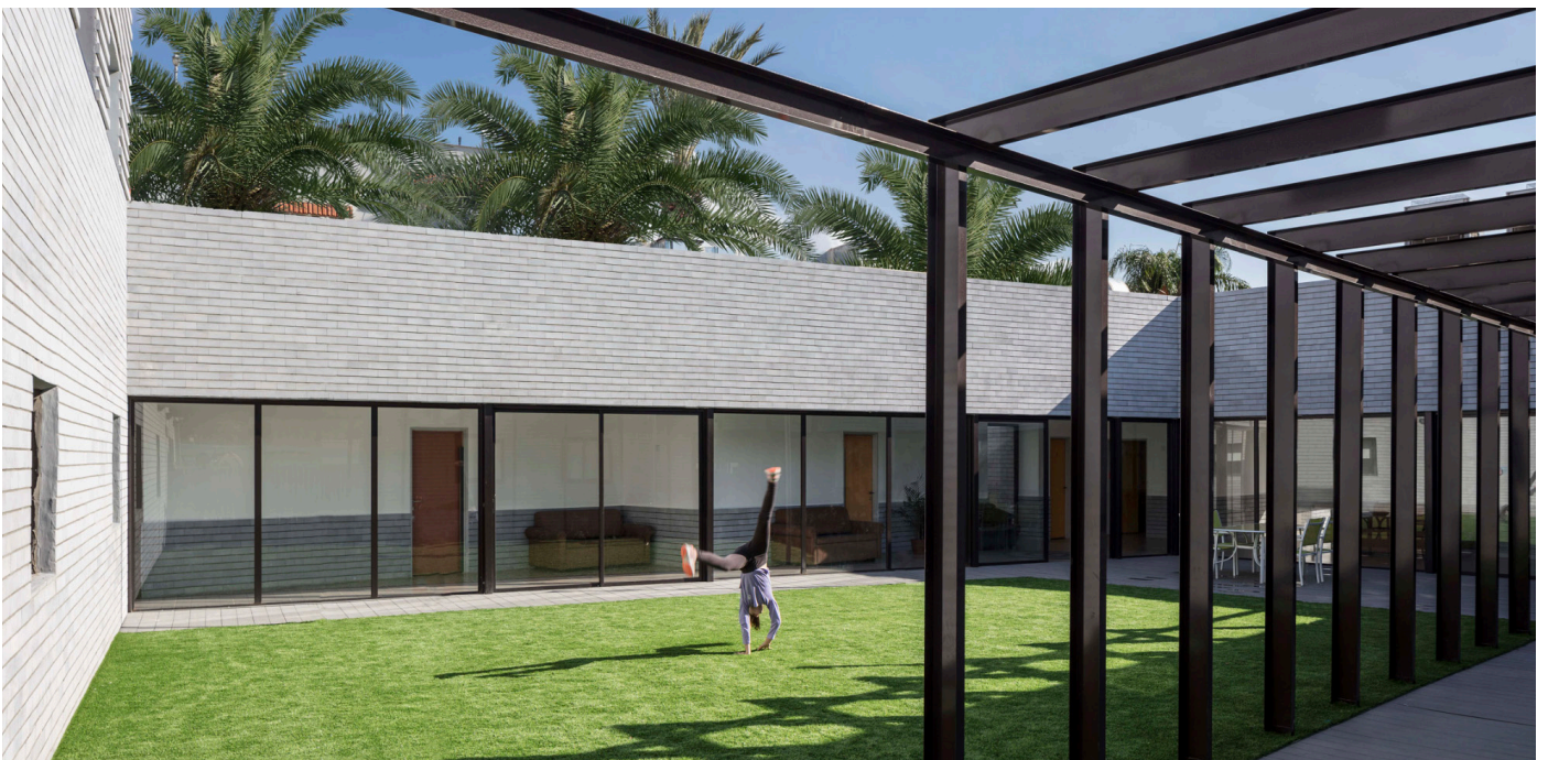
Figure 9. Shelter for Victims of Domestic Violence, Tel Aviv, designed by Amos Goldreich Architecture. Courtyard exterior view. (Stephenson and Geron, 2018)
