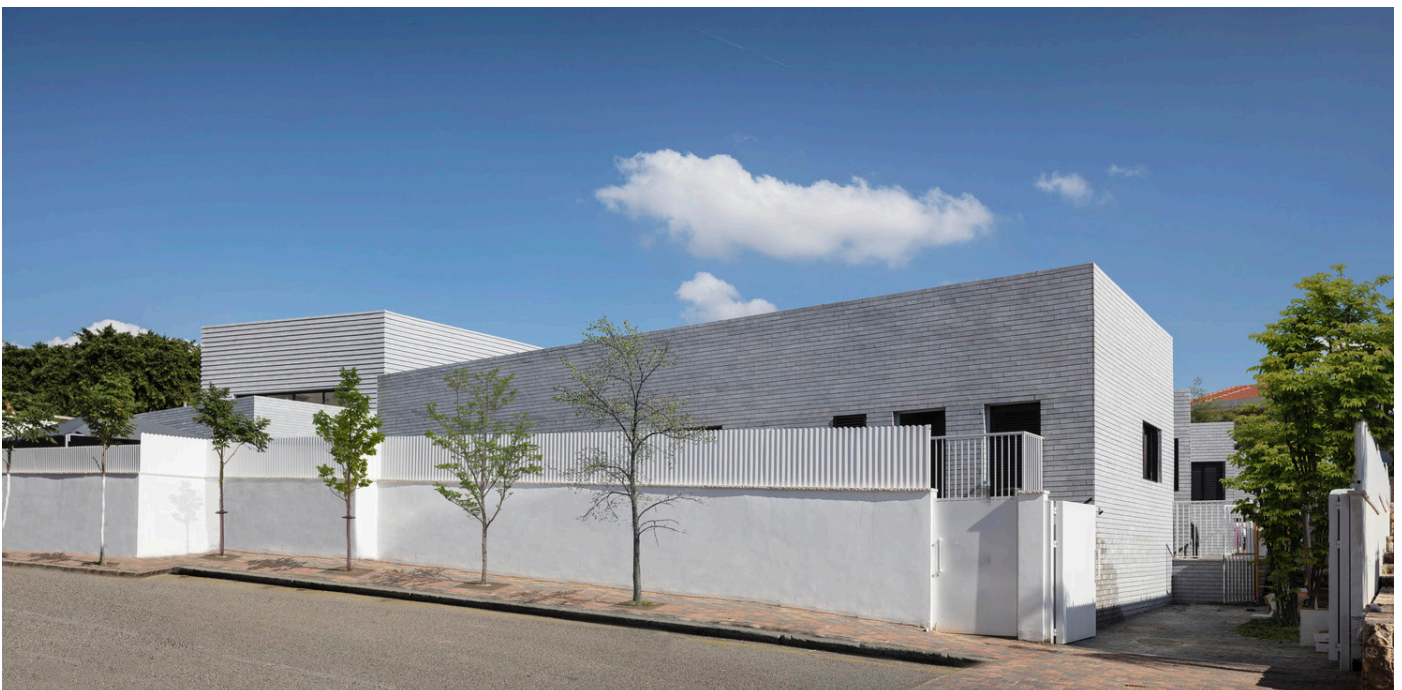
Figure 7. Shelter for Victims of Domestic Violence, Tel Aviv, designed by Amos Goldreich Architecture. Exterior view showing the entrance and façade designed to ensure privacy and safety. (Stephenson and Geron, 2018)
