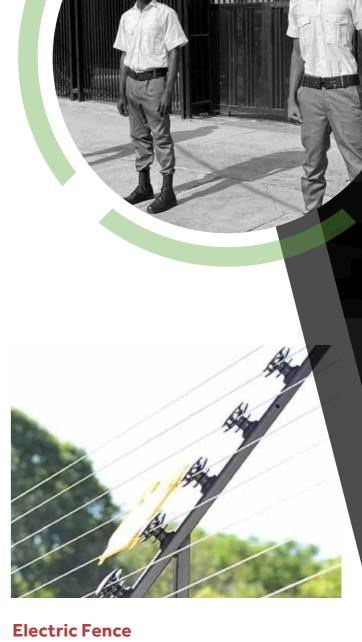
The Electro-Fence™ is a programmable intelligence system. It is capable of triggering an alarm when the preset conditions are met. The duration of the high voltage pulses a mere fraction of a second. This makes the system non-lethal, but powerful enough to incapacitate an intruder. That is why the perimeter intruder detection system is referred to as a non-lethal security fence system.
