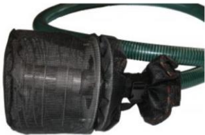
Installed Screen over Existing Suction Hose and Strainer
