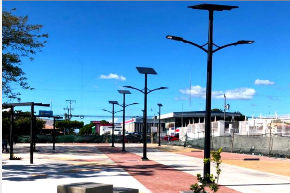
Utah, US Project
