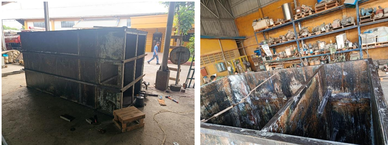
Existing septic tanks and site condition before project implementation
