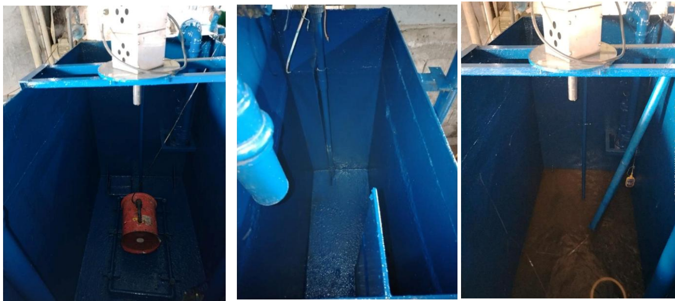
During installation and commissioning
