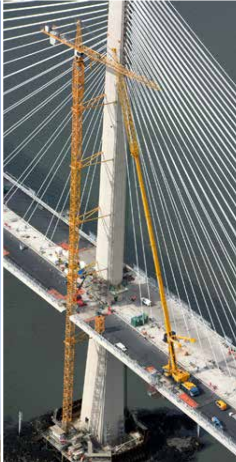
▲ Constructing the Queensferry Crossing.
