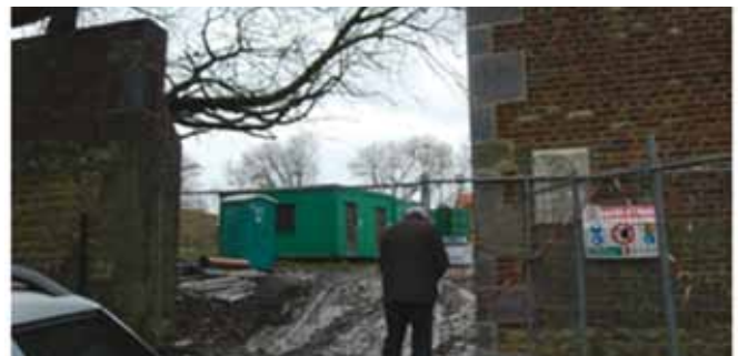
The piers of the north gate repaired & ready to receive the new gates. January 2015.
