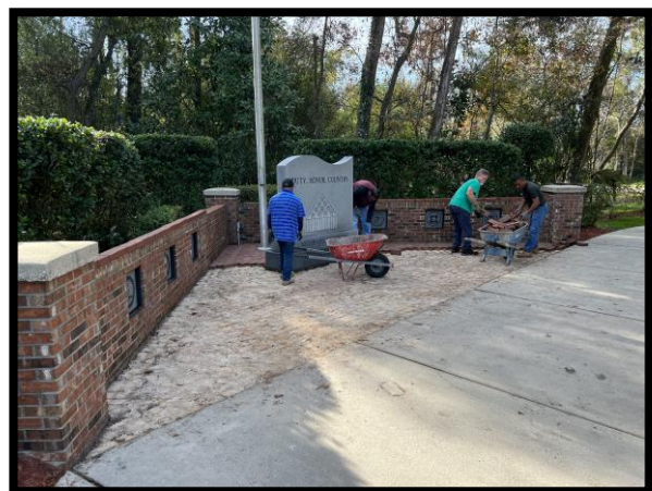
Removal of existing pavers
