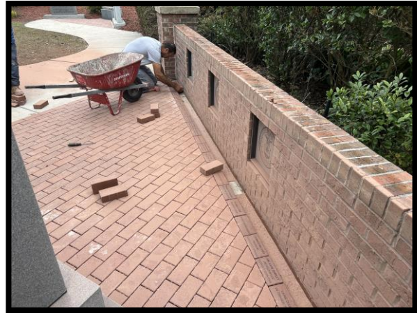
Installation of new pavers
