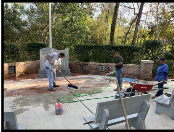
Placement of sand between the new pavers
