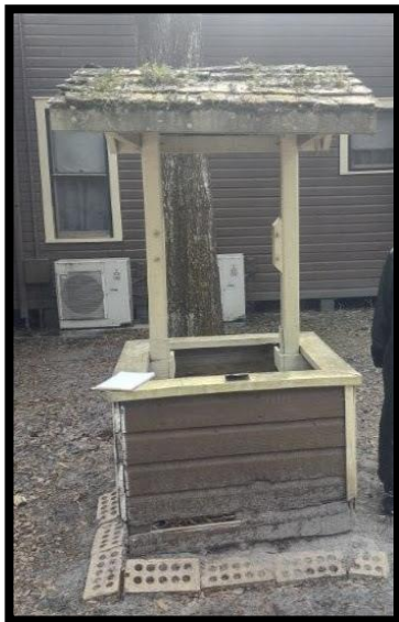
Well-house prior to rehabilitation
