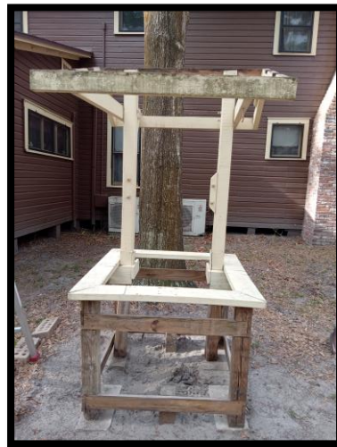
Well-house during rehabilitation
