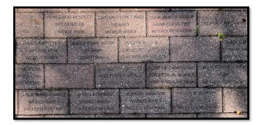
During Phase 1 for this issue, a search was begun to identify a new provider for the pavers that would hold up better in our temperature and moisture conditions. We have received sample engraved pavers that we believe will be better suited for the exposure that we have to expect. We are now in Phase 2 of resolving this issue. The committee must individually review the installed pavers to determine which have to be replaced and then contract with the manufacturer to provide these engraved pavers.
