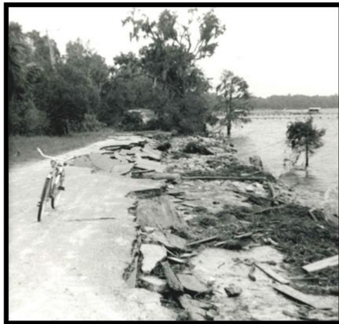
Damage to River Road in Orange Park
