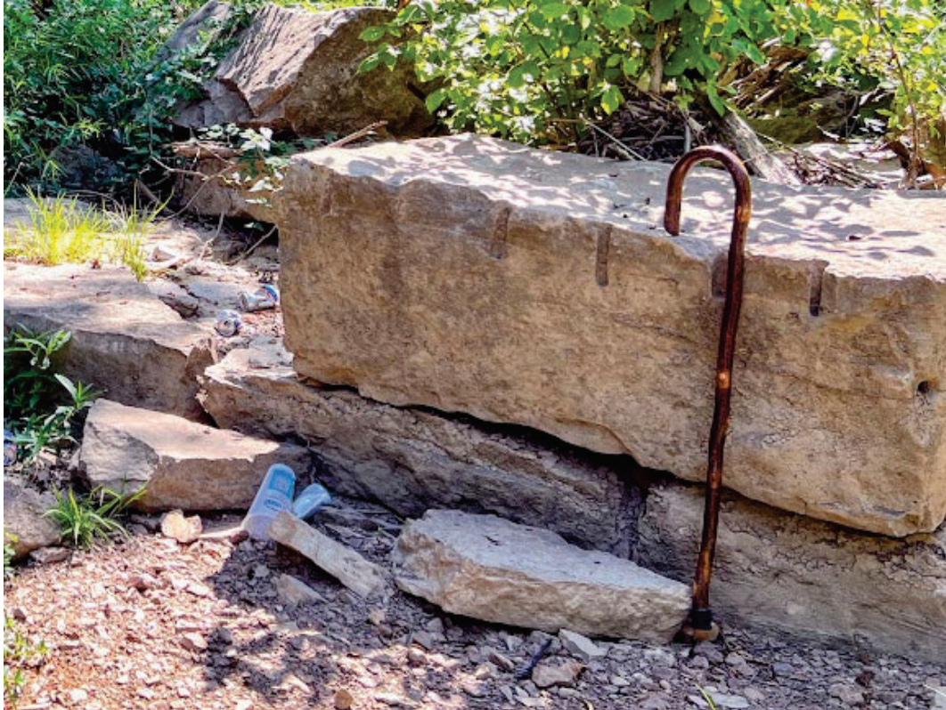
In a photo taken July 21, 2022, while the river is low shows the rough stone blocks of the dam with the hand hammered drill marks to quarry the stone. My cane is approximately a yard from base to the top of the bend. This stone must weigh tons.
