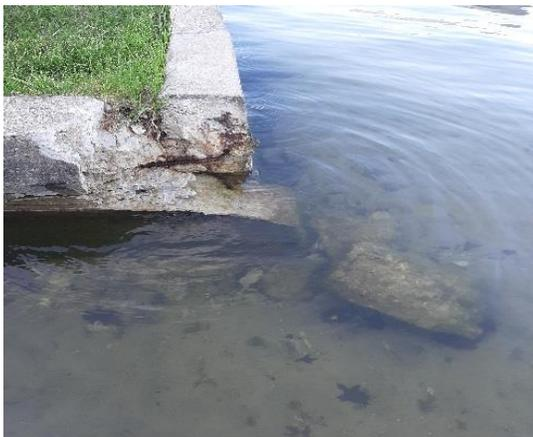
This was damage to a concrete seawall on Woodbeck Lake caused by boaters speeding by too close to shore.
