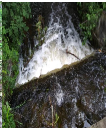
Water flow cleared
