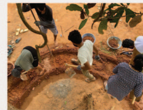
Excavated About 6" Deep.
