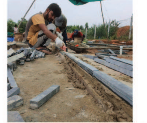
Waste kadapa stones where used to make secondary plinth
