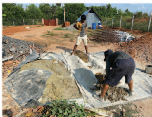
Making lime mortar 1:4
