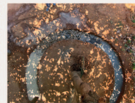
Thin layer of limecrete over granite aggregate.
