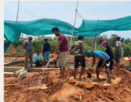
Preparing mud plaster
