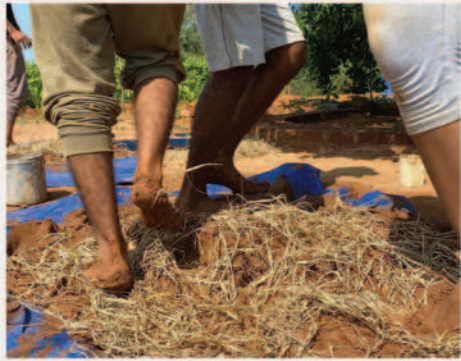
Mixing Straws with Mud
