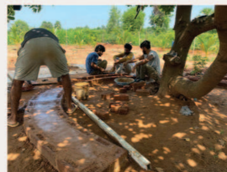
The Brick Surkhi is compacted & the surface is given a rough finish
