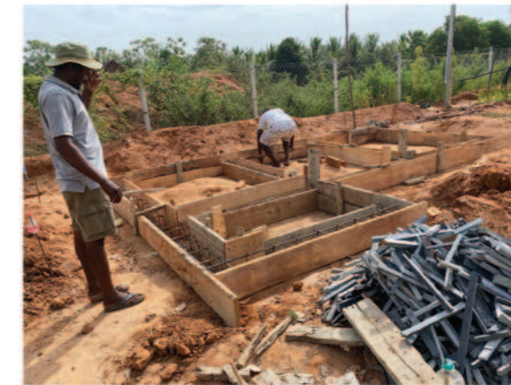
Plinth beam formwork
