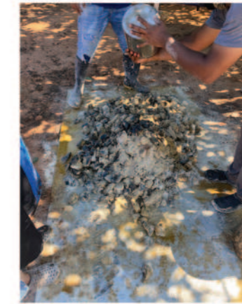
Coarse aggregate mixed with lime
