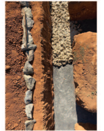
Foundation filled upto 2" of coarse aggregate.
