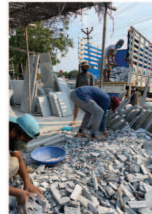
Salvaging waste granite material
