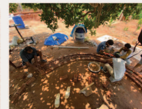
Center is filled with surkhi
