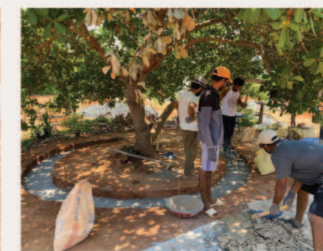
Laying a course M-sand & Aggregates
