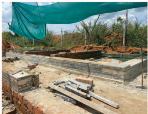
9" Stone Masonry Work
