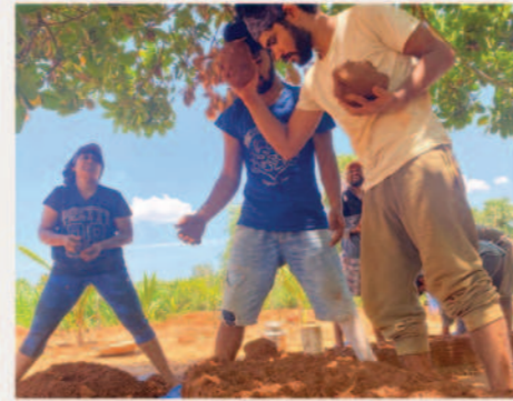
Laying the cob
