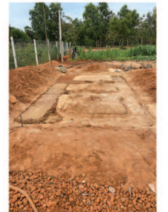
Final fine layer of plc-foundation
