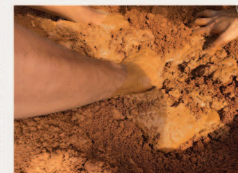
The Brick Surkhi is compacted & the surface is given a rough finish
