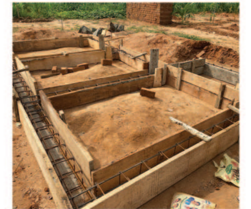
Plinth beam formwork
