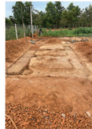
Foundation completed with PLC
