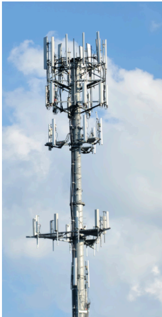
Above photographs purchased via Canva. Left: monopole macro cell tower. Top right: sector/panel antennas on building. Bottom right: multiple antennas affixed to smokestack, acting as a “stealth” macro cell tower).
