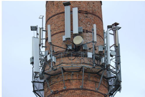
Above photographs purchased via Canva. Left: monopole macro cell tower. Top right: sector/panel antennas on building. Bottom right: multiple antennas affixed to smokestack, acting as a “stealth” macro cell tower).
