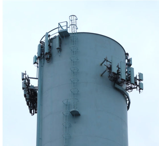
Left: Smokestack, corner of Park St and Prospect, 2074 Park St, Hartford, CT. Right: Water tower in Manchester, CT. Wireless equipment is often painted to camouflage its appearance. Photos by R. Stephens.
