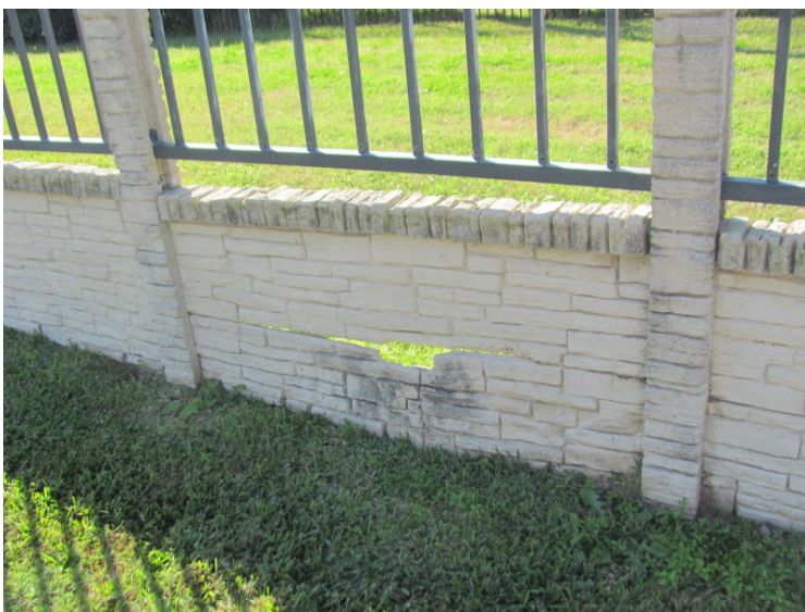
Damaged concrete panel
