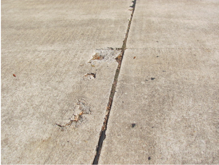
Concrete deterioration at Tall Canyon Drive
