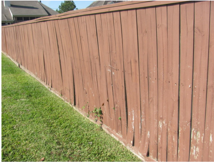
Warped boards at wood fence along Canyon Gate Boulevard near Marina Canyon Way
