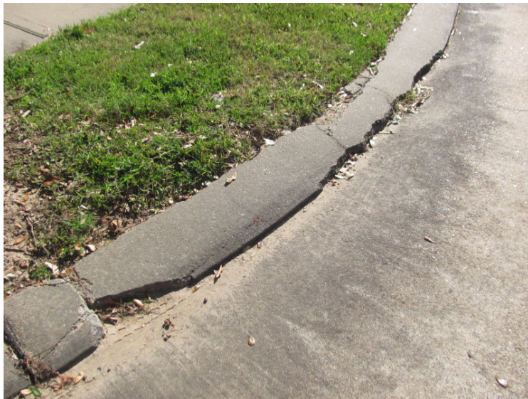
Damaged and spalled concrete curb
