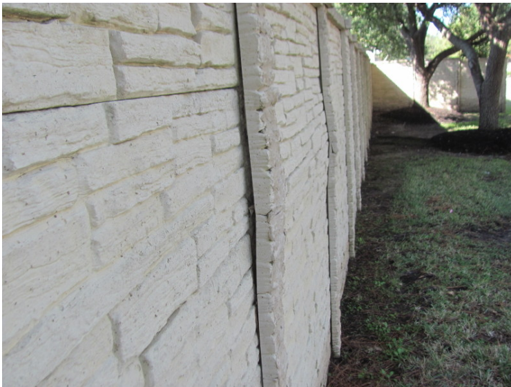
Movement evident at wall
