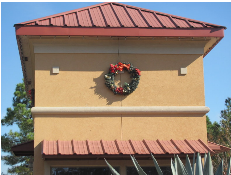
Corrugated metal roofing at guard house
