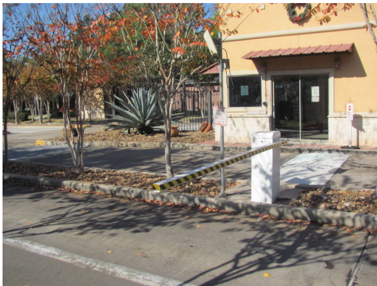
Gate operator and swing arm
