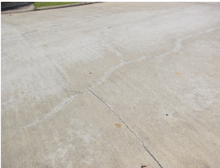
Concrete cracks at Canyon Park Drive
