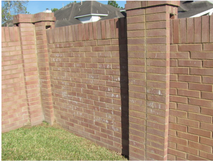
Efflorescence
