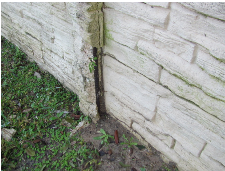
Concrete post deterioration and exposed reinforcement
