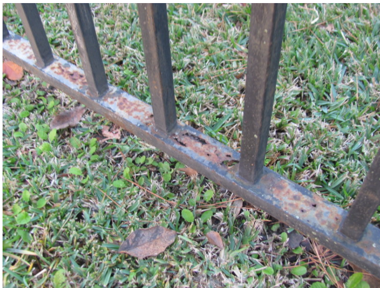
Corrosion at steel fence
