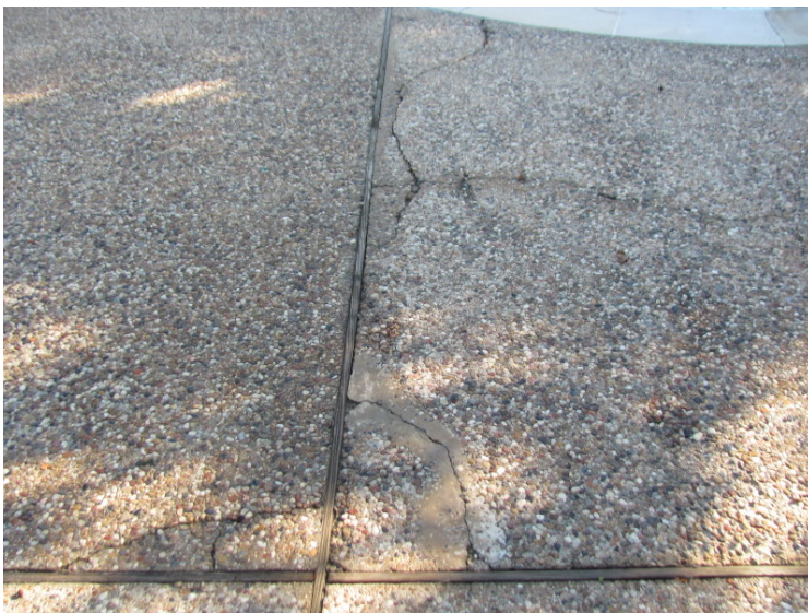
Concrete cracks at pool deck
