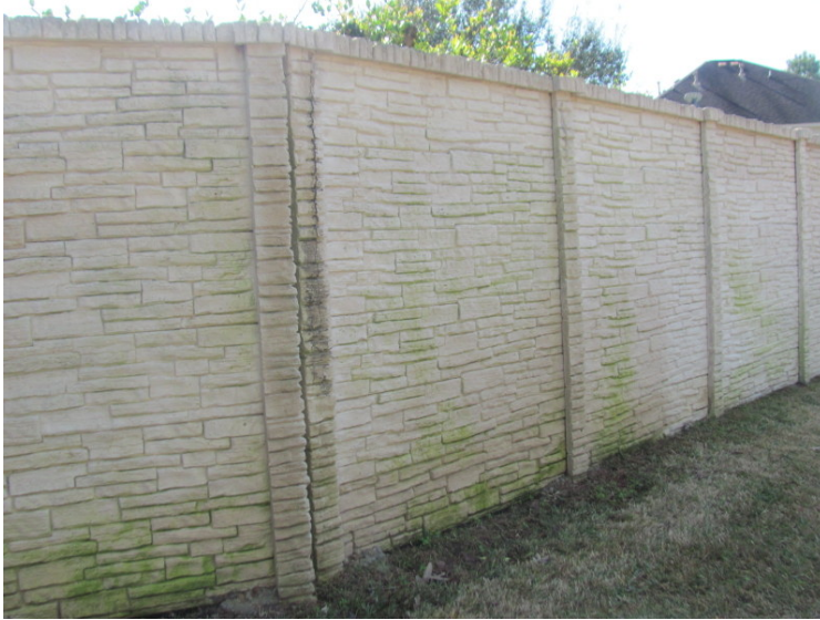
Stains at panelized concrete wall
