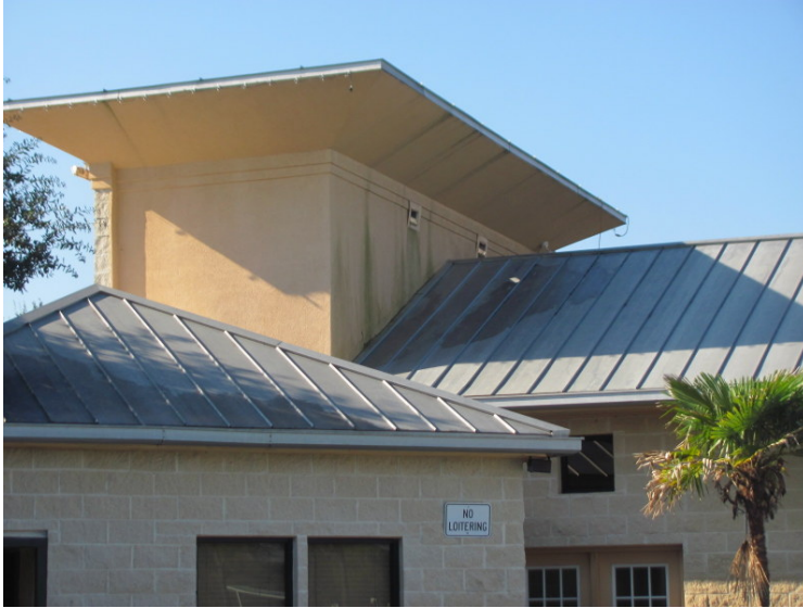
Standing seam metal roofing at clubhouse
