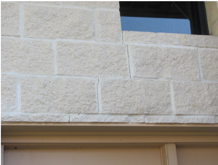
Masonry step crack at clubhouse
