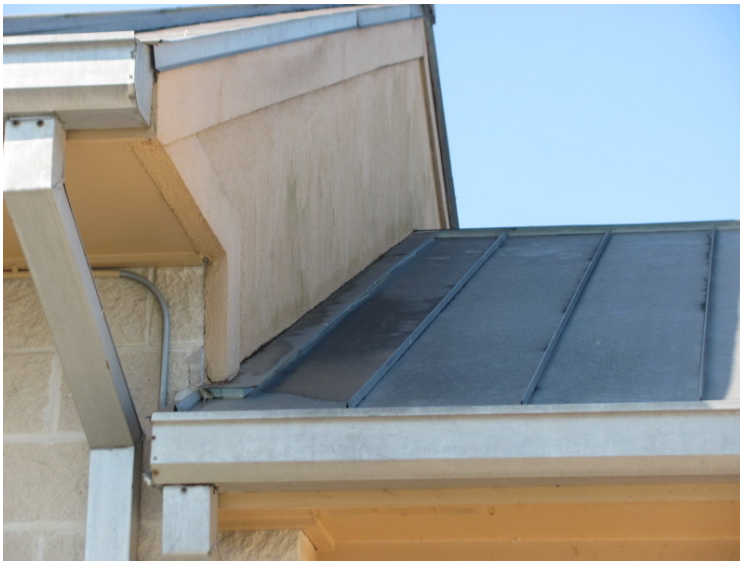
Stains and finish deterioration at clubhouse
