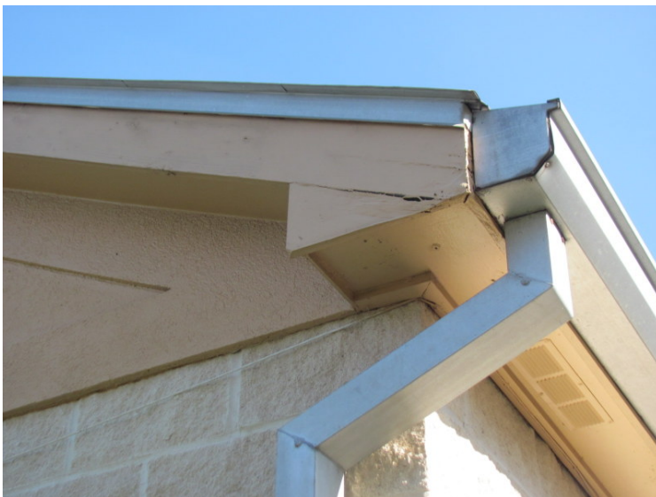
Minor wood deterioration at clubhouse
