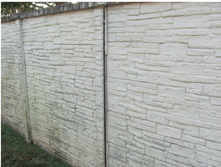
Concrete post deterioration and exposed reinforcement
