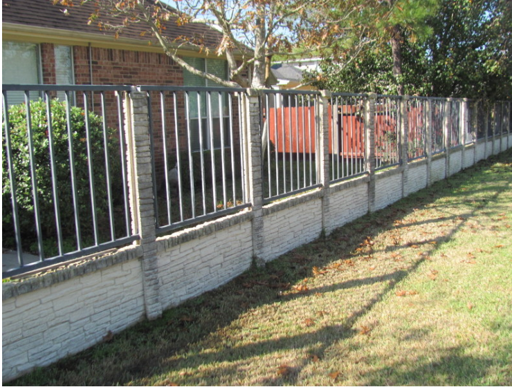
Panelized concrete wall with steel fence
