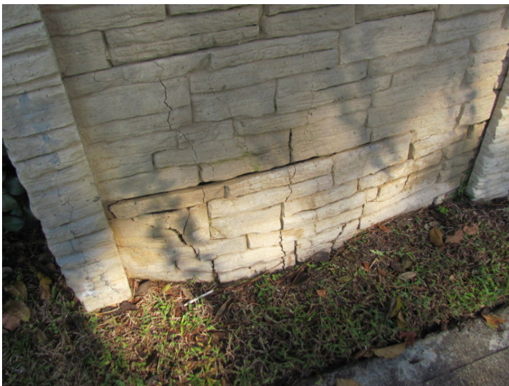
Shifted and cracked concrete panel
