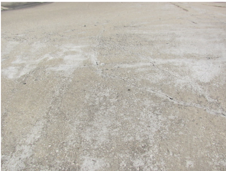
Concrete cracks and spalls at Canyon Park Drive
