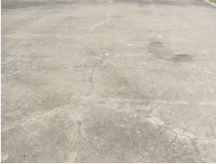
Concrete cracks at open basketball court near skate park
