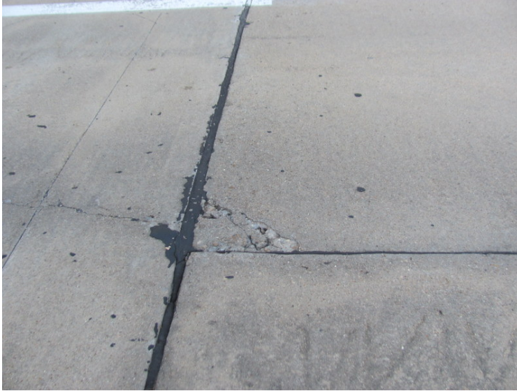
Concrete cracks near joint
