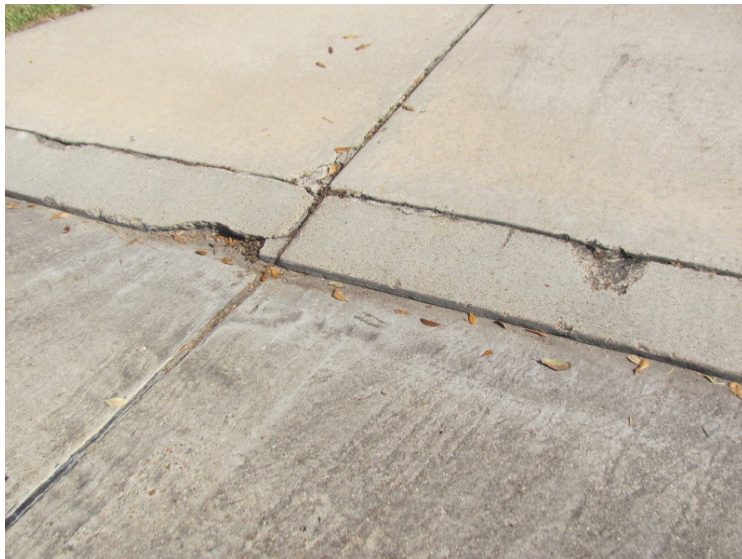
Damaged and spalled concrete curb
