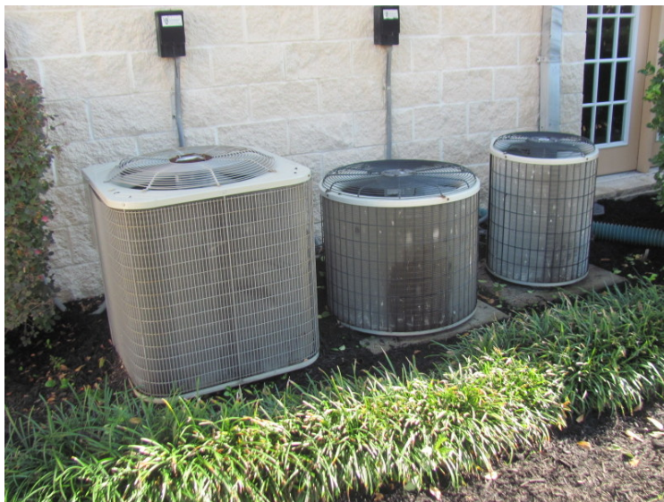
Split system condensing units
