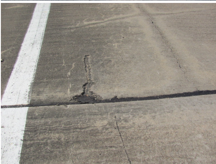
Concrete damage at Canyon Gate Boulevard
