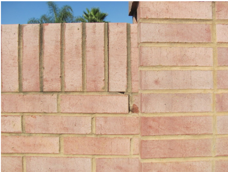
Mortar deterioration
