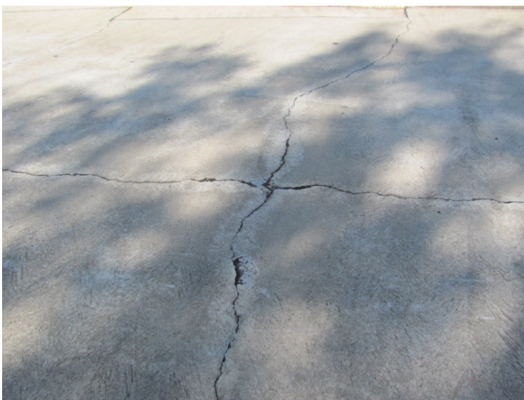
Concrete cracks at Canyon Gate Boulevard
