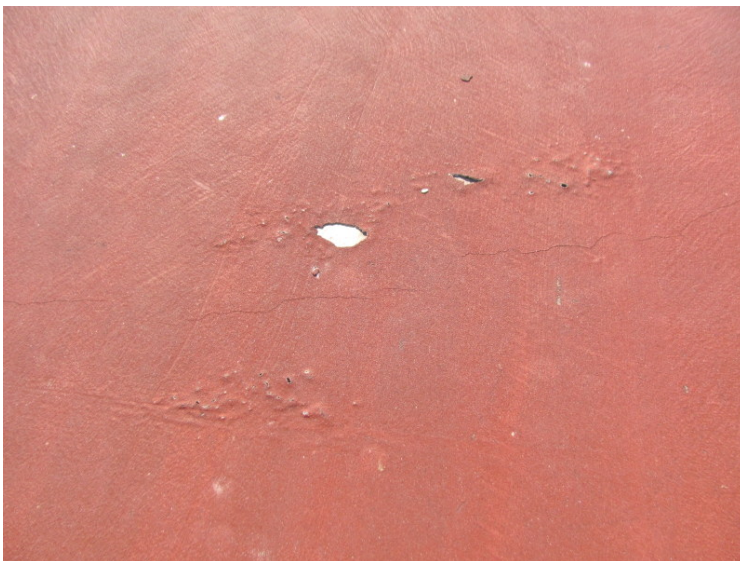
Blistered and chipped color coat at tennis court
