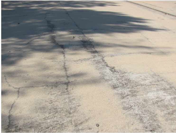
Concrete cracks at Wind Canyon Drive
