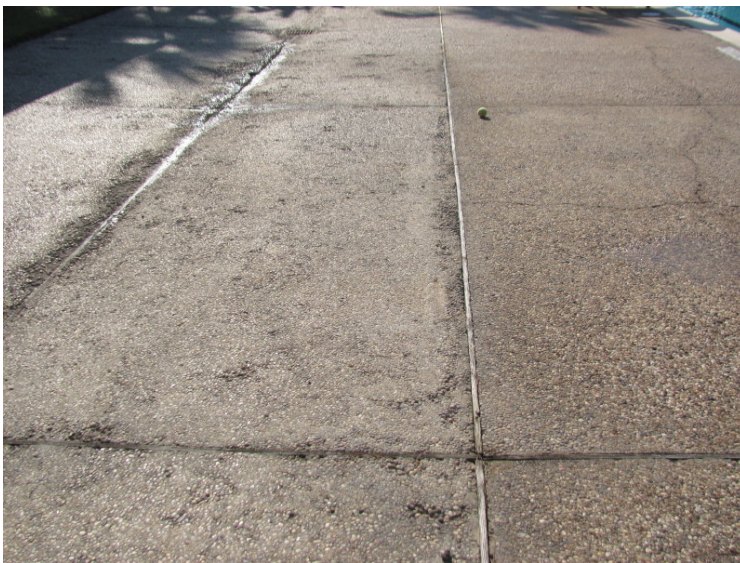
Concrete cracks and spalls at pool deck
