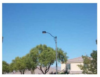
An allowance for Street Light Repair has been included in the Study to be done as needed. The Street Lights are not supported properly. Complete replacement has not been included in the Study. Further evaluation is recommended.
