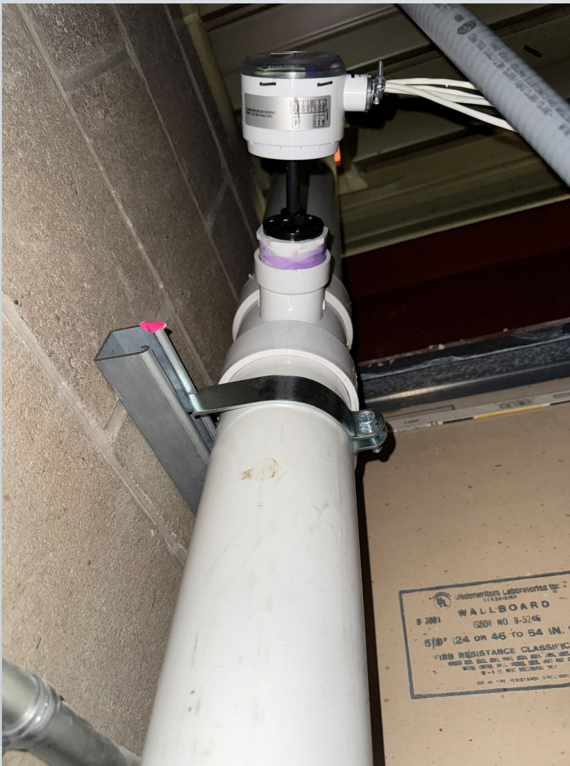
View of CFM Sensor mount installed in a 2" Schedule 40 PVC Tee.
