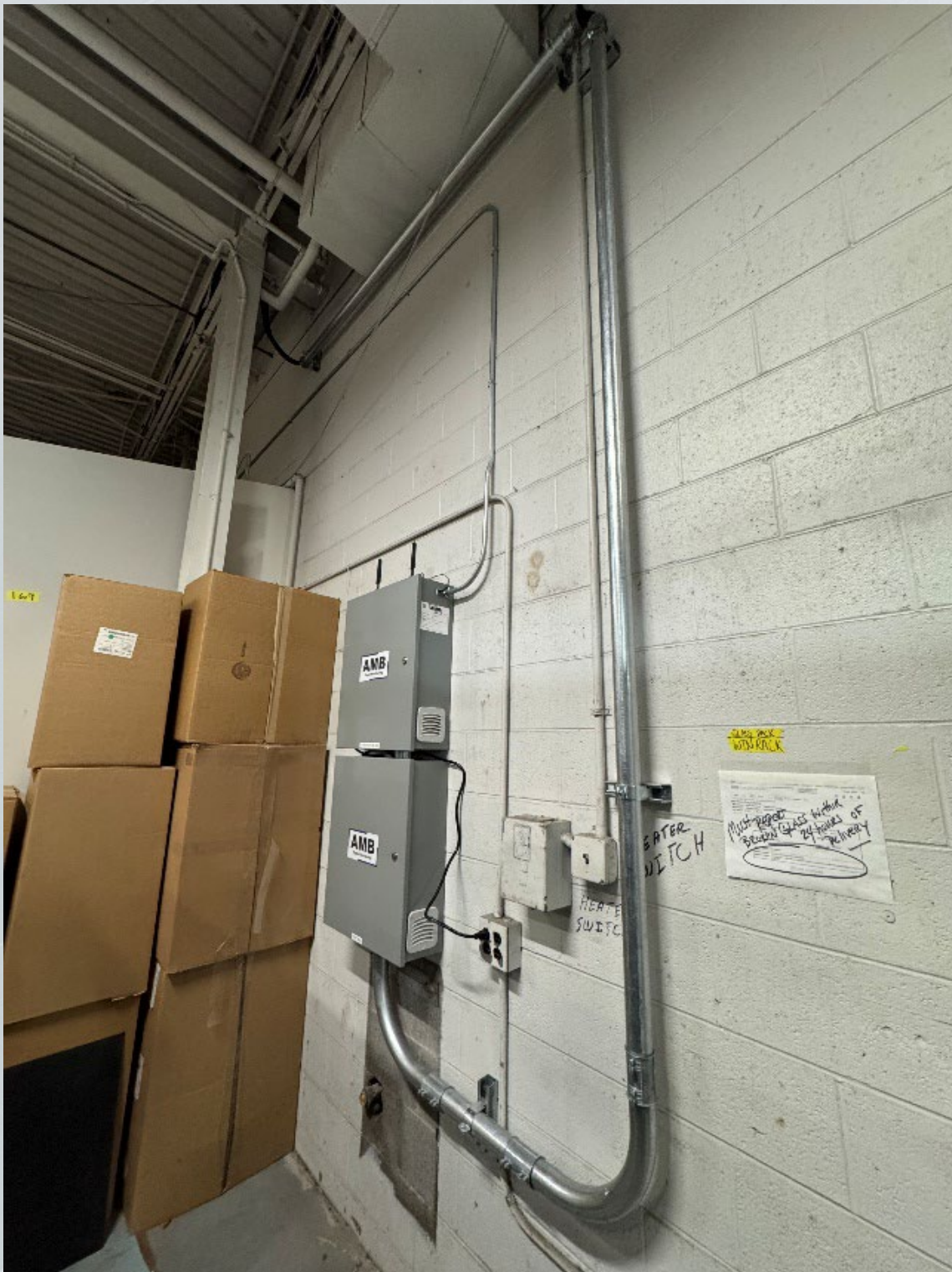
View of CFM Sensor wire within conduit entering the top right corner of the wall mounted communication box.
