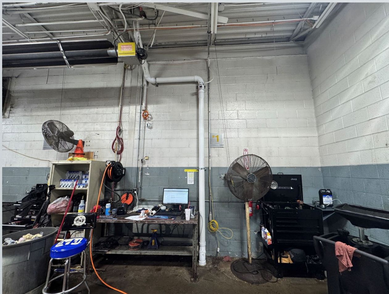
View of CFM Sensor installed on vent riser.
