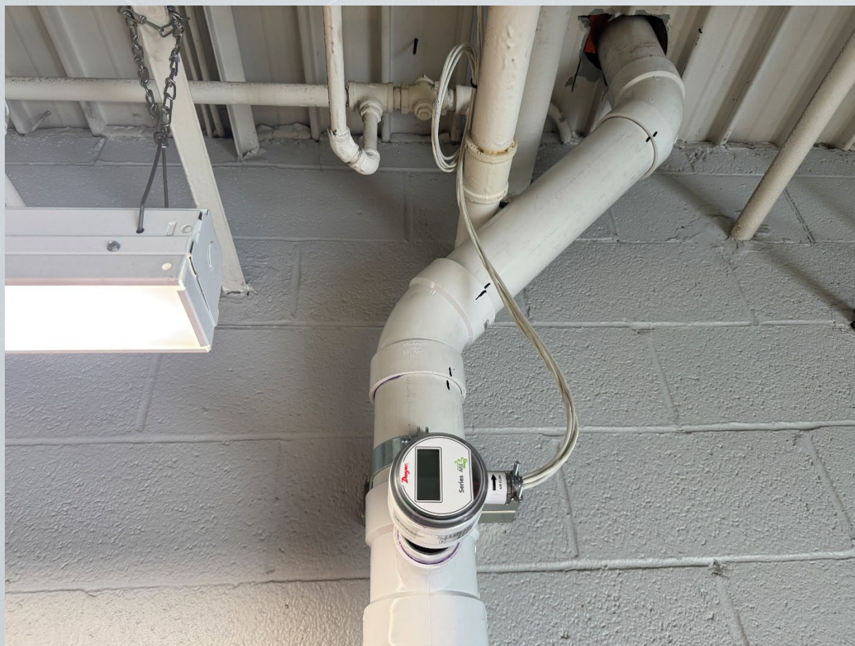
View of CFM Sensor installed on vent riser with low voltage power wire and communication wire.
