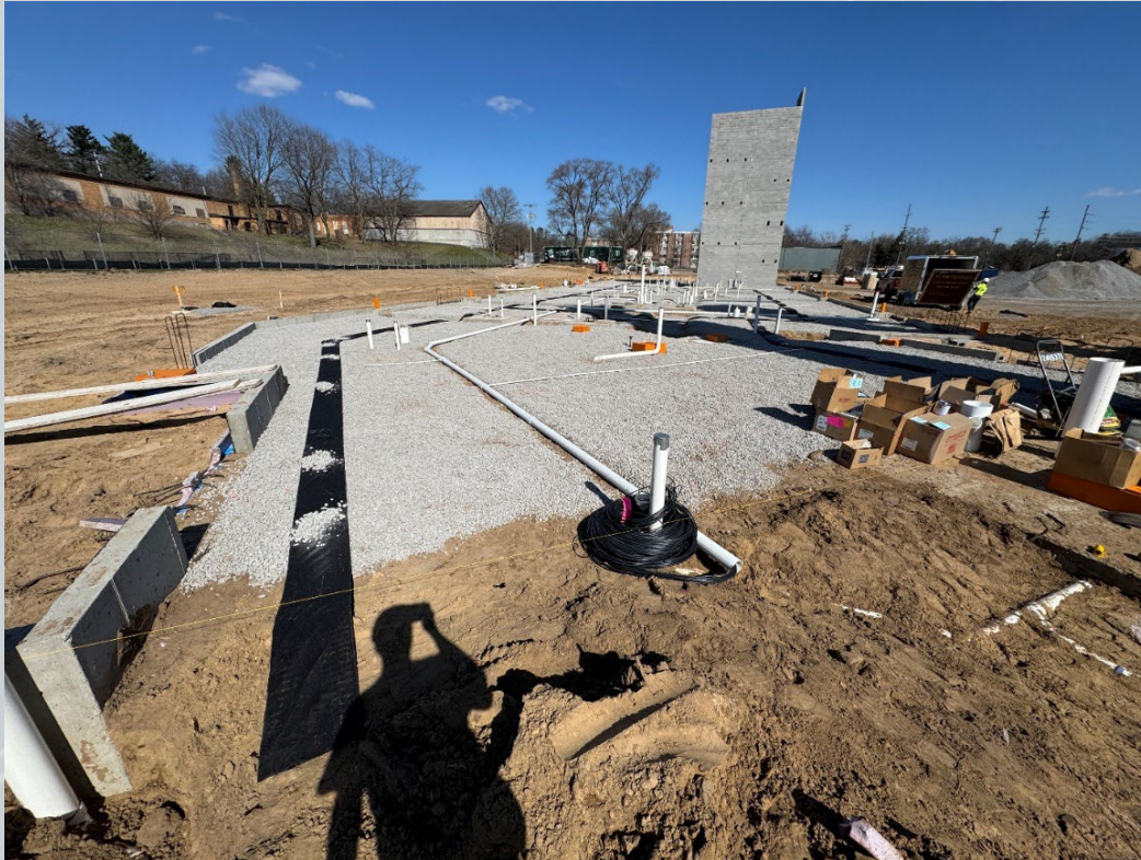
View of tubing within the PVC conveyance pipe.
