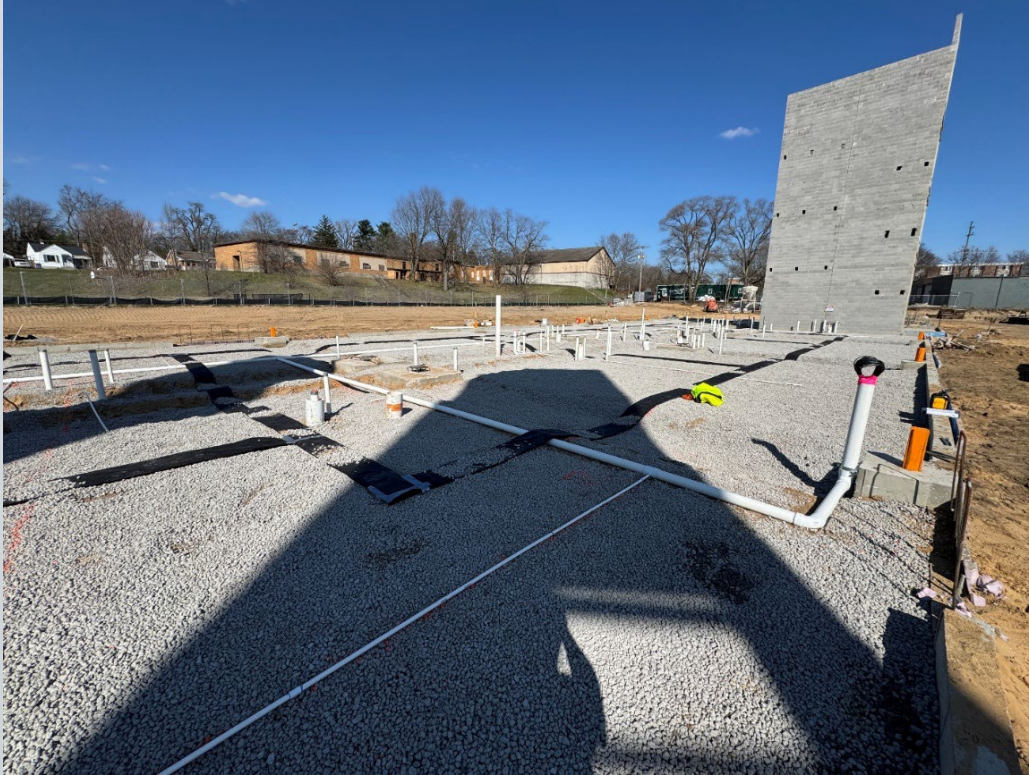
General view of installed below slab pressure test ports, pressure test port tubing, and PVC conveyance pipe.
