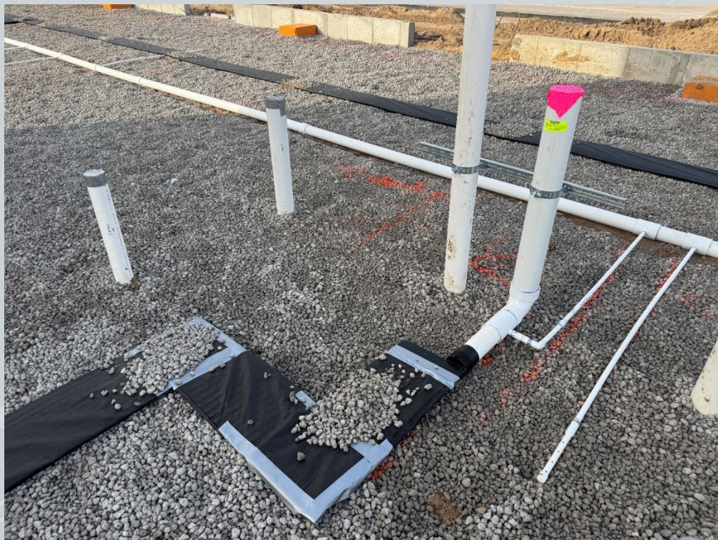
View of vent riser pressure test port and below slab pressure test port connected to PVC conveyance pipe.
