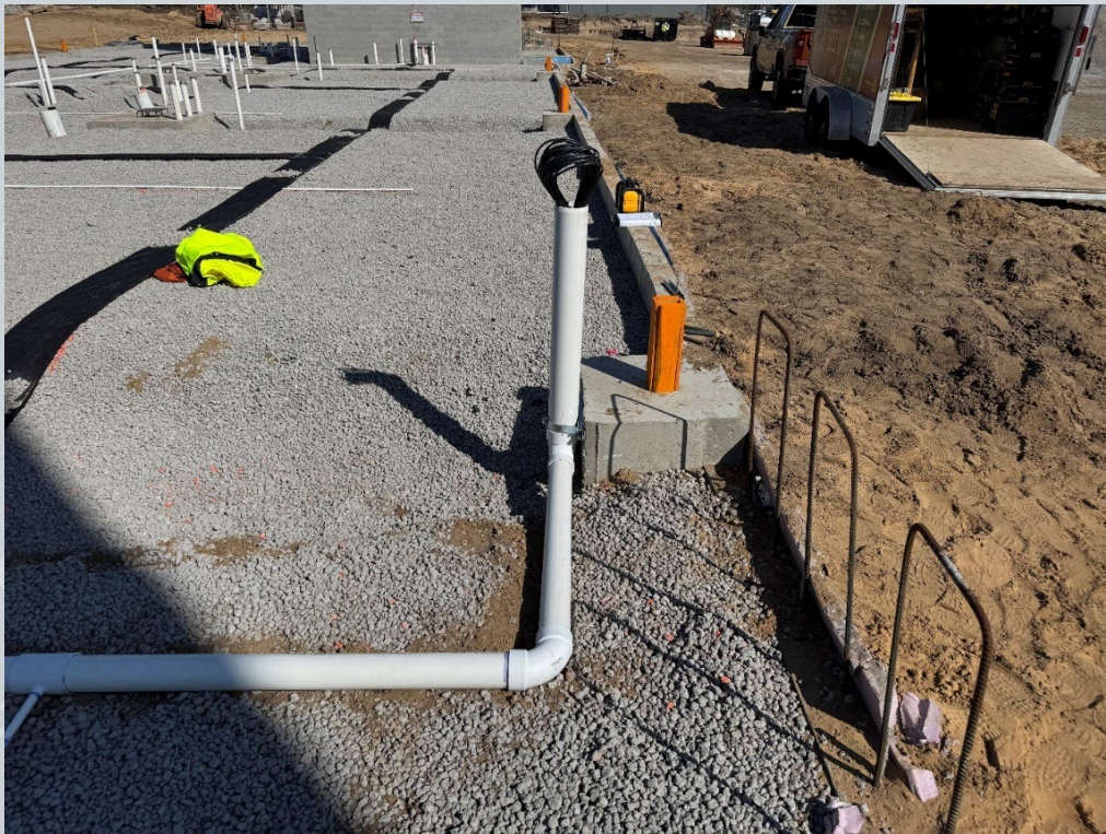
View of stubbed up pressure test port tubing for wall boxes.
