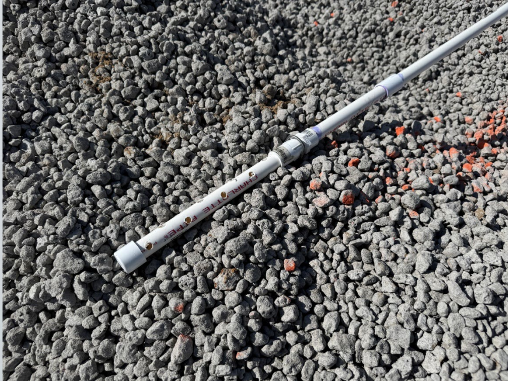
View of below slab pressure test port connected to ½" Schedule 40 PVC.
