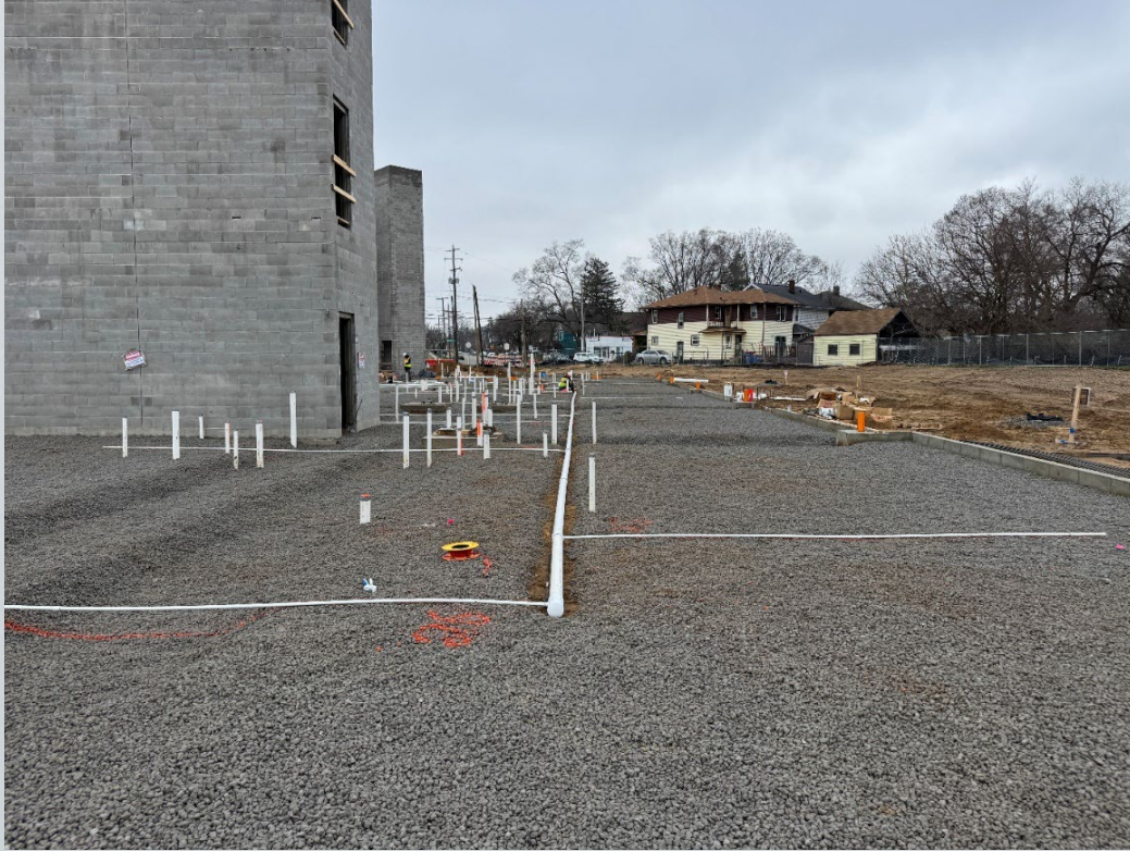
View of below slab pressure test ports connected to PVC conveyance pipe.
