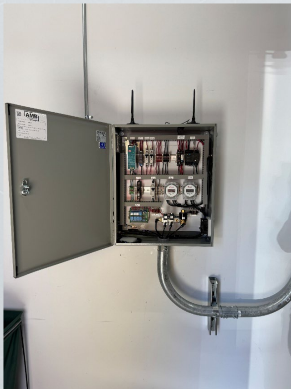
View of pressure test port tubing connected to solenoids inside of the port box.
