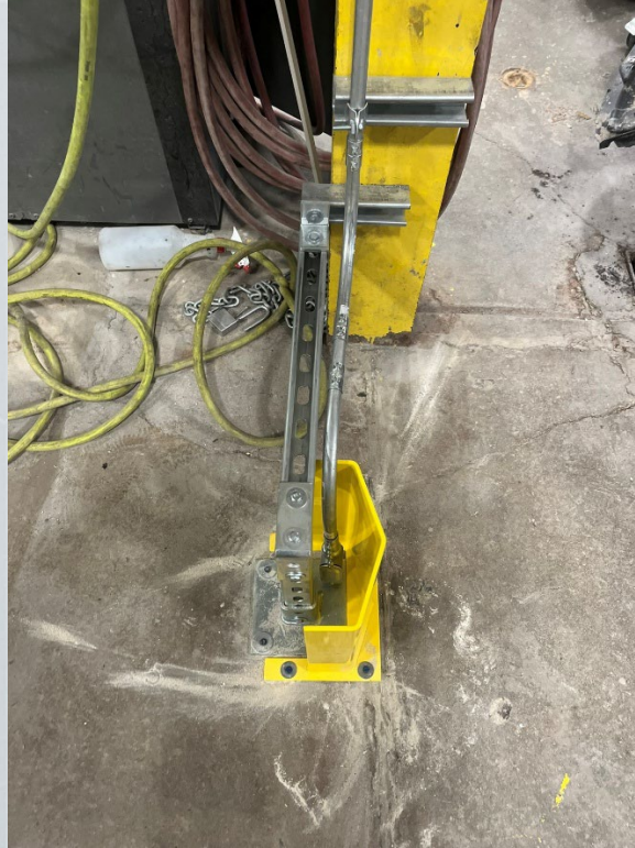
View of installed above slab pressure test port in strut base.
