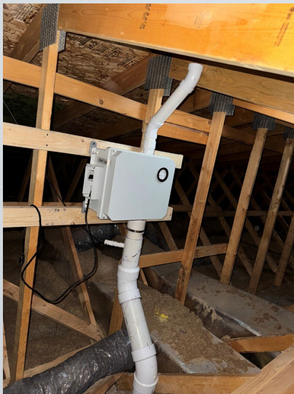
View of installed vent riser pressure test port.
