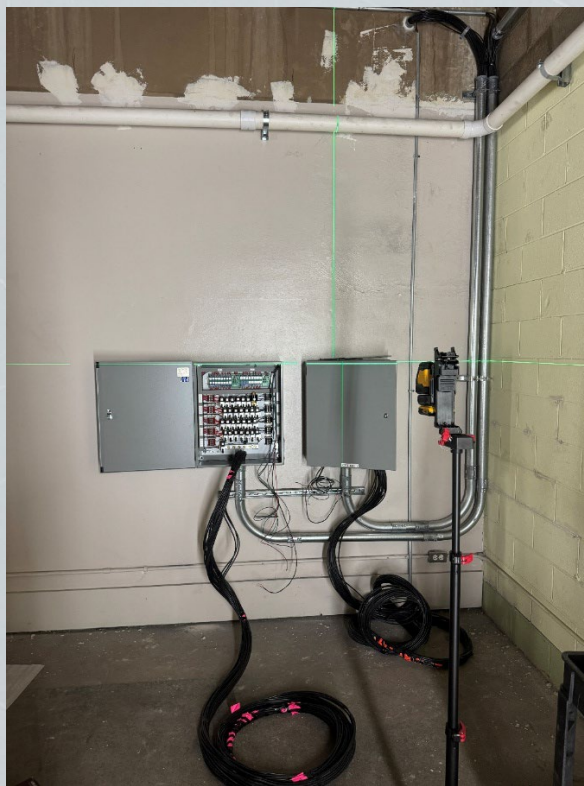
View of installed port boxes with labeled tubing to be connected to solenoids.
