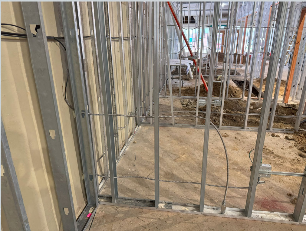
View of installed above slab pressure test port within a wall of a remodel protected with flex conduit. Also view of pressure test port tubing running back to the wall box location.
