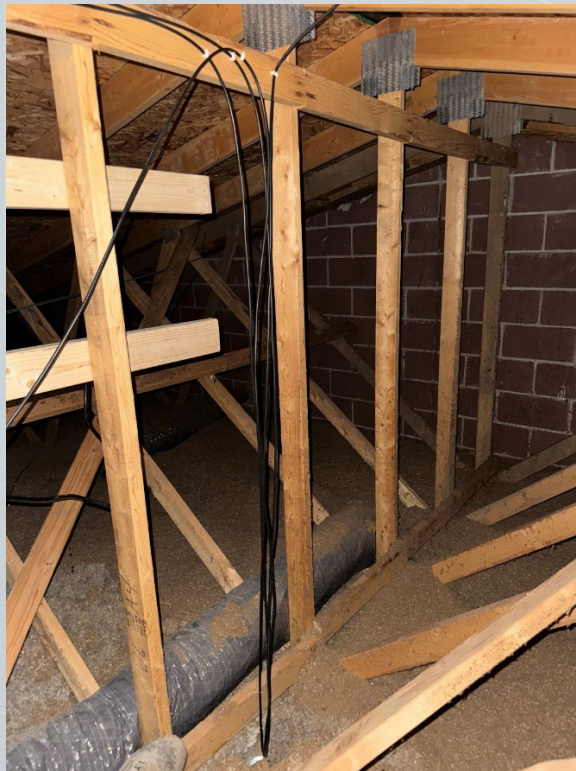
View of routing pressure test port tubing down to the wall box location.
