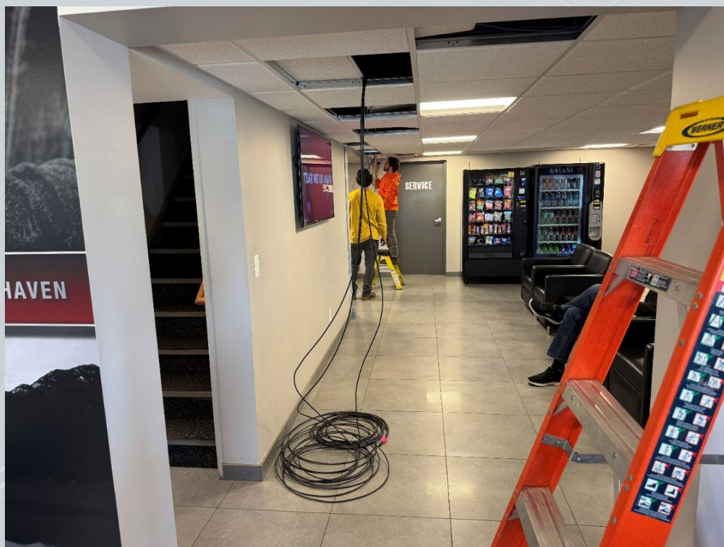
View of routing pressure test port tubing above drop ceiling.
