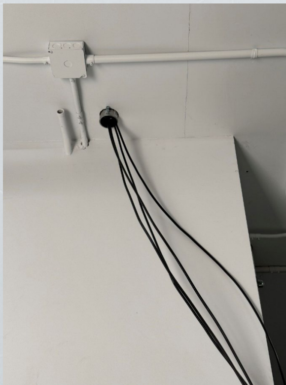
View of pressure test port tubing coming down from the attic.
