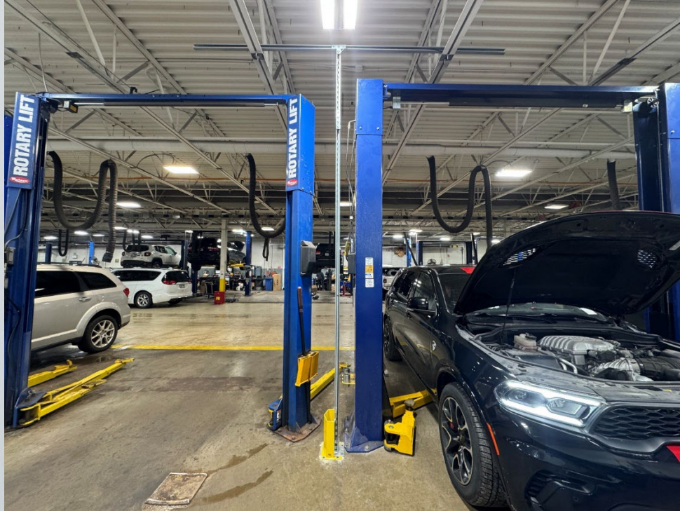
View of installed above slab pressure test port using unistrut as support when there is no wall or column present.
