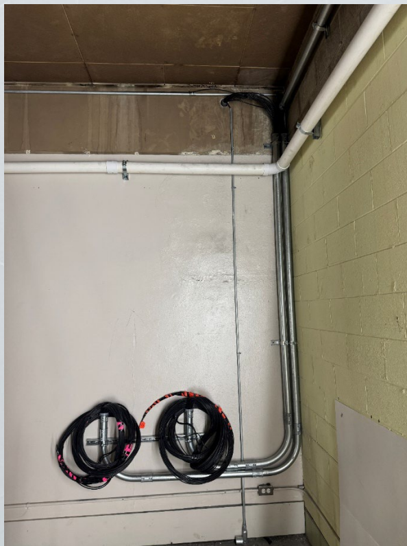
View of stubbed up pressure test port tubing for a telemetry system with two port boxes.
