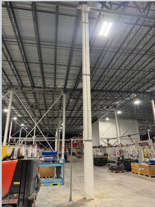
View of installed above slab pressure test port along column on warehouse.
