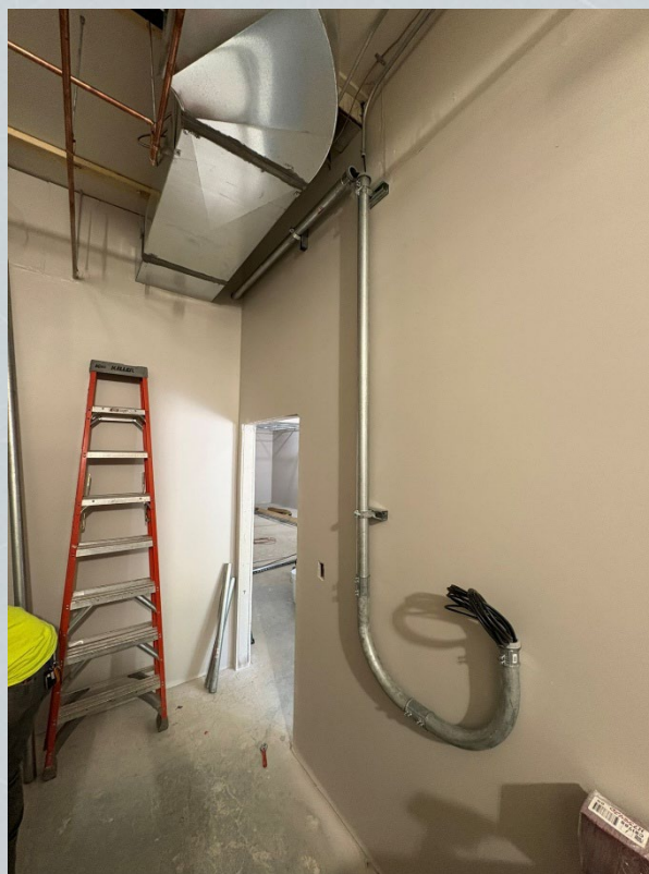
View of stubbed up pressure test port tubing for wall box.
