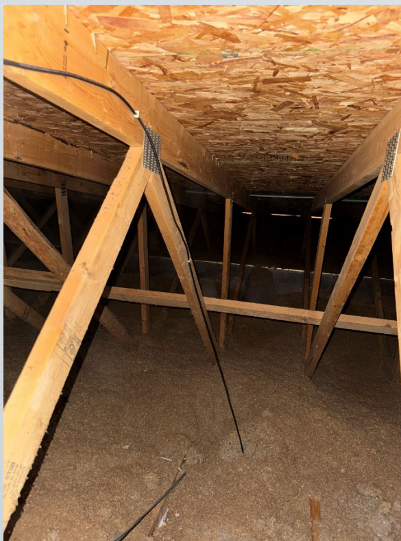
View of routing pressure test port tubing down to above slab pressure test port.
