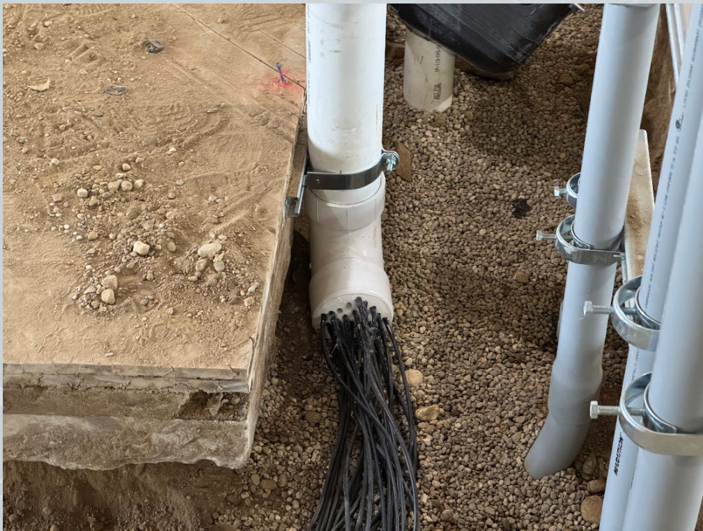
View of pressure test port tubing going into 4" PVC Stub up. Silicone is used to seal around the tubing going into the 4" cap.
