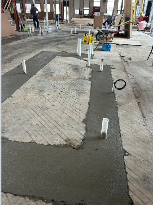
View of a vent riser pressure test port tubing stubbed up for a vent riser not placed in trench.
