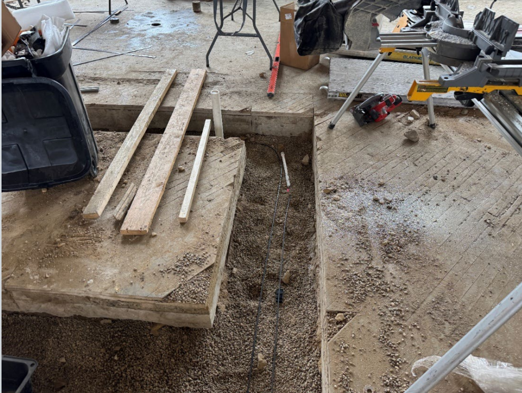
View of below slab pressure test port and tubing in trench.
