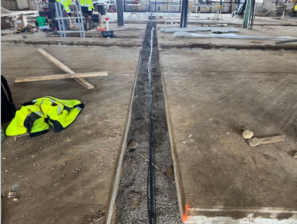
View of pressure test port tubing in trench.
