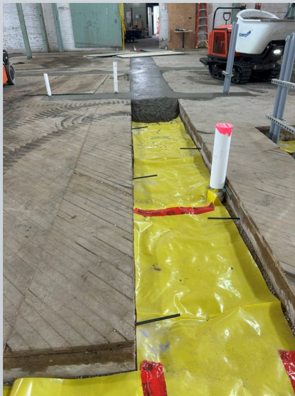
View of plastic placed in trench to protect tubing and below slab pressure test ports.
