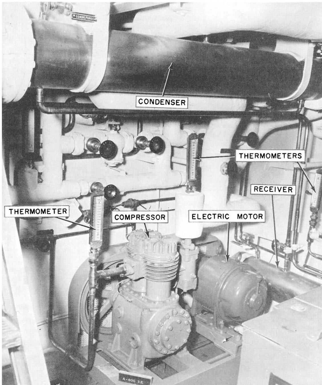
Figure 11-2.—High-pressure side of R-12 installation aboard ship.
