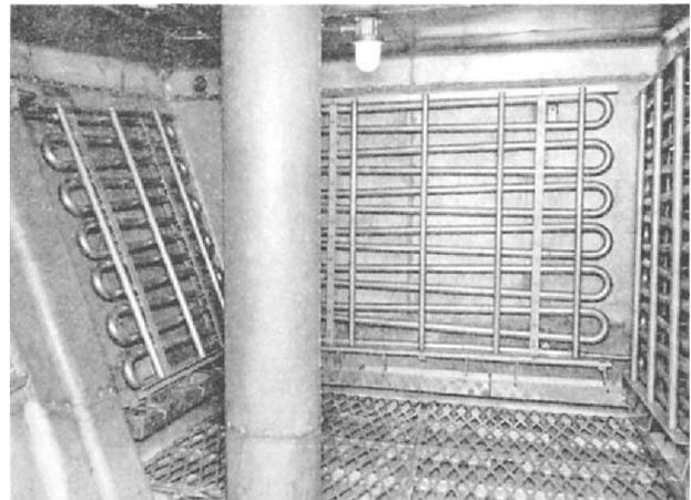
Figure 11-4.—Evaporator tubing.
