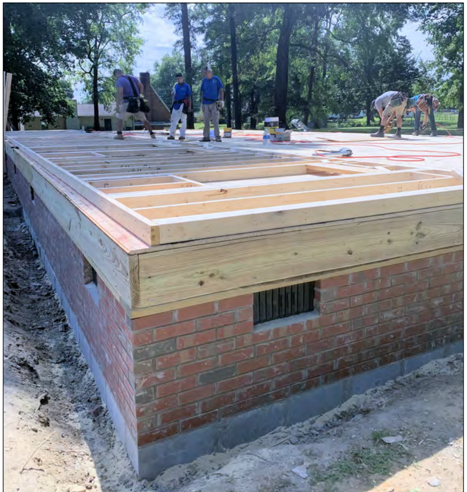
Above: The brick foundation is in, the floor is in, and workers were preparing to erect the exterior framing for the front of the new building when this photo was taken. Below: The trusses for the roof of the new building are all stacked up ready for installation once the framing of the new building is completed. The new building will be “dried-in” when the foundation is complete, the exterior framing is up, windows and exterior doors are installed and the roof is sheathed with water-resistant material. (Photos by Kevin Jones)
